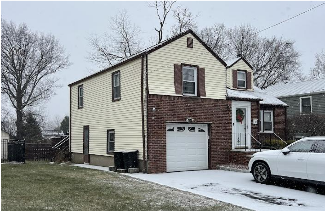
Figure 2: Front yard of 10 Shrump Place from the northwest corner of the property
