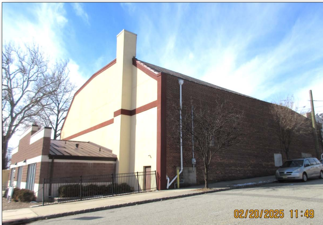
Photo 2: View of the northern side of the subject property from the northeast on Erwin Place.
