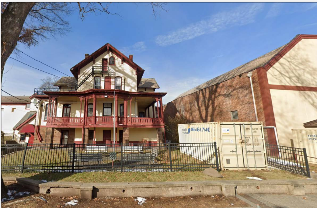
Photo 4: View of the subject property with the West Orange Community House abutting it to the south.
