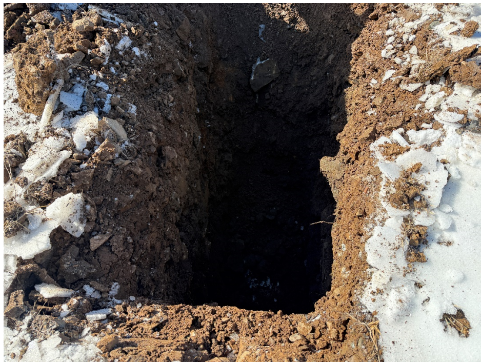
Photo 3: Test Pit TP-11
