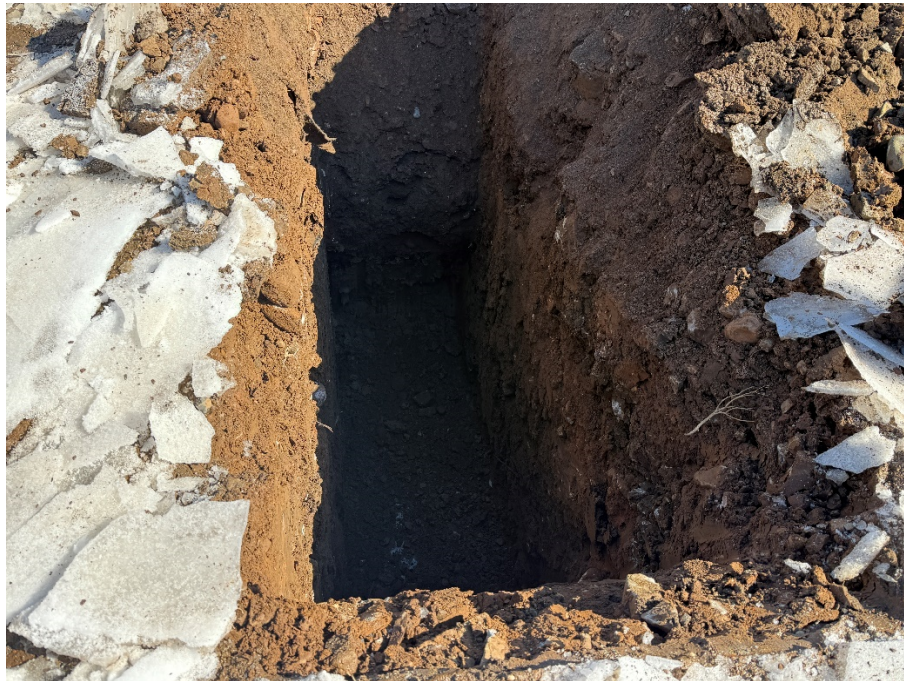
Photo 1: Test Pit TP-01
