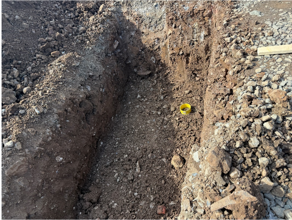
Photo 2: Infiltration test at Test Pit TP-03
