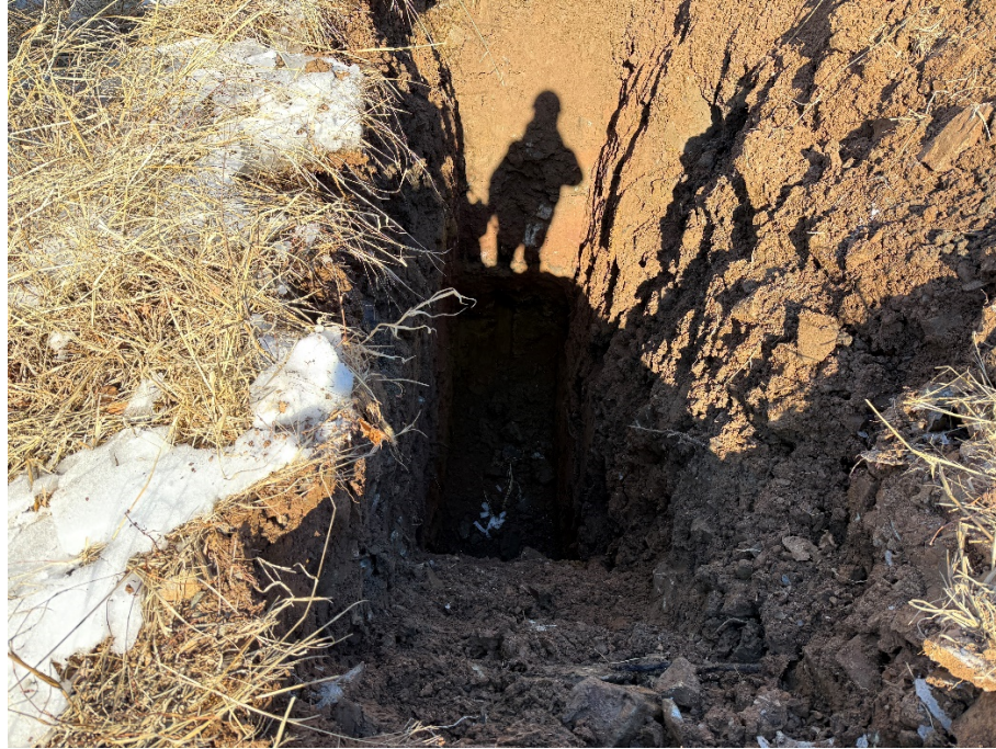
Photo 4: Test Pit TP-12
