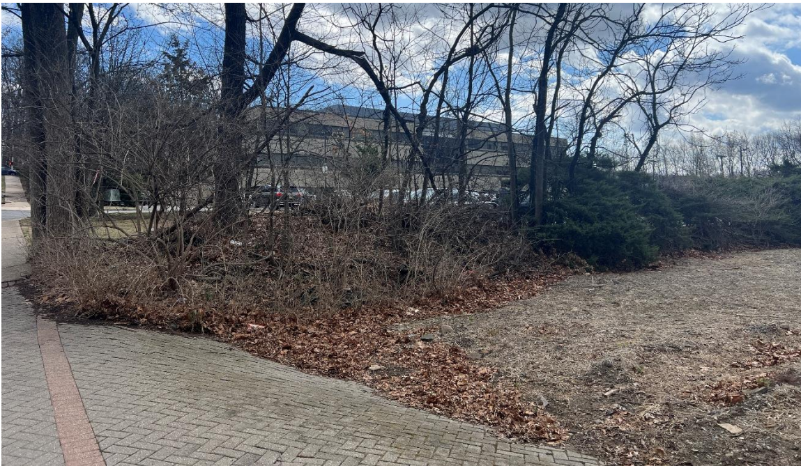
Figure 8: Rear of the office building to the east
