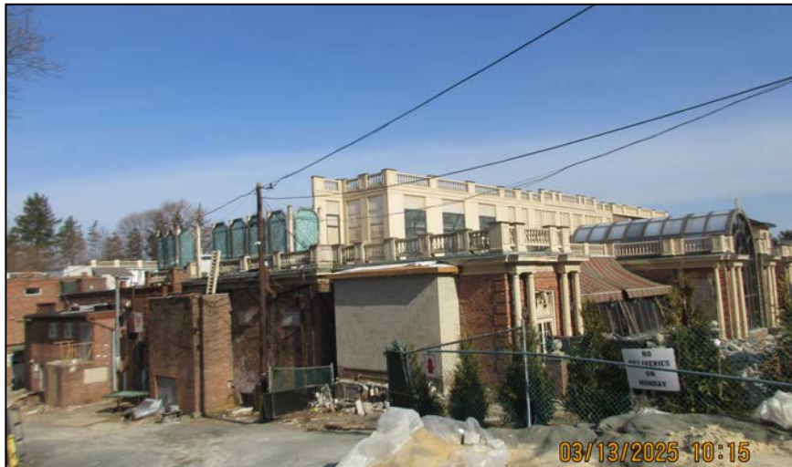
Photo 5: View of the southern façade of the main building.
