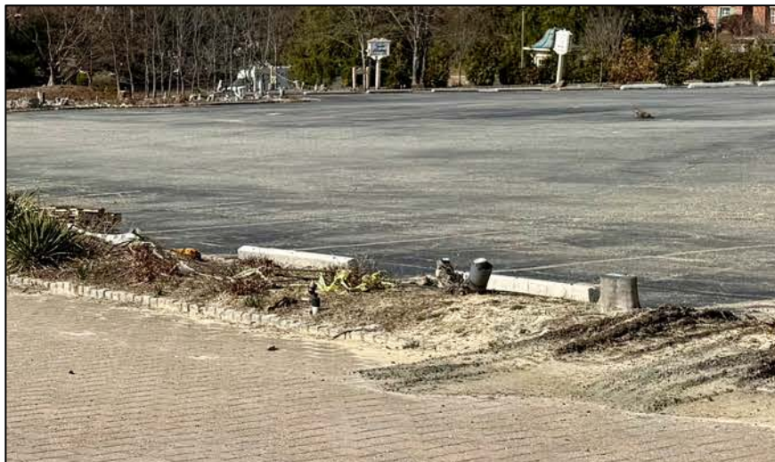
Photo 2: View looking to the northwest across Lot B showing some of the stumps from the trees that were previously cut down.
