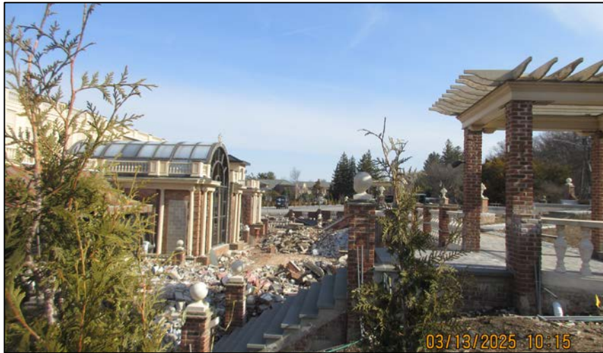
Photo 4: View of the courtyard between the elevated garden area to the right and the front façade of the main building to the left. The courtyard will be built up to the level of the 1 st floor of the main building.
