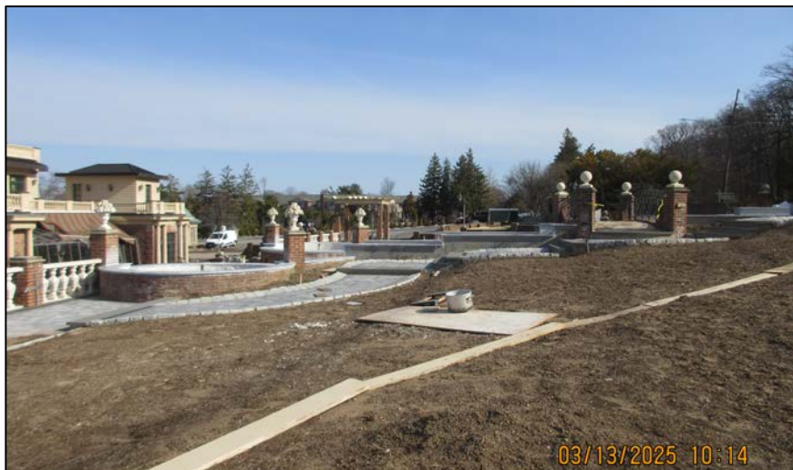
Photo 3: View looking north across the elevated garden area located at the front of the main building.
