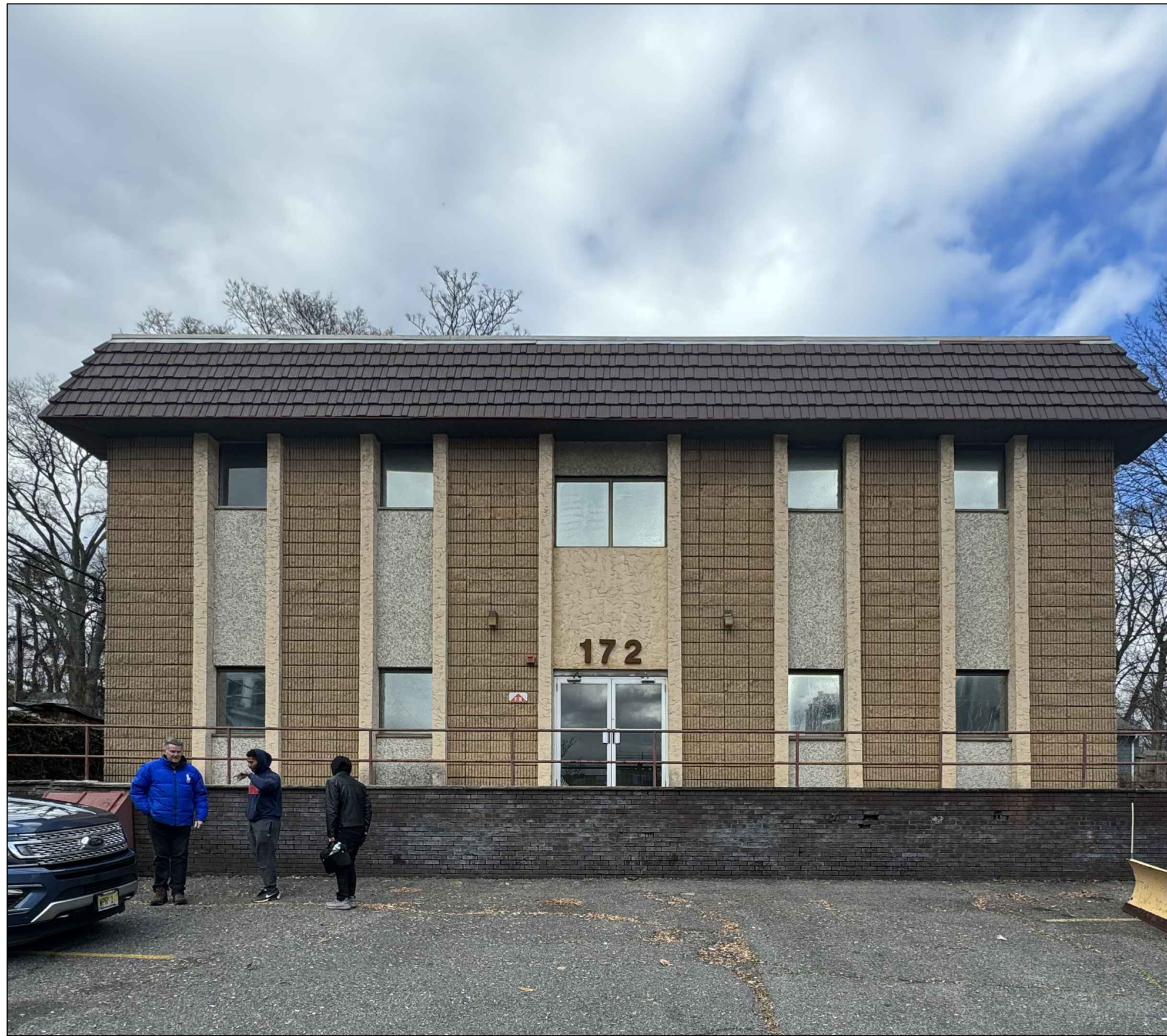
EX EXISTING PHOTOGRAPH NO TO SCALE
