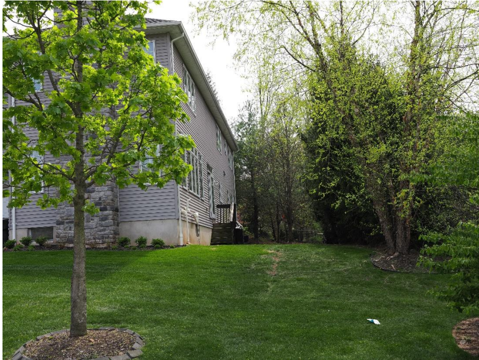
Figure 4: 7 Himsl Court - looking into rear yard setback
