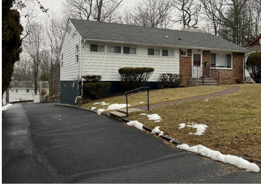
Figure 2: View of 77-79 Lessing Road
