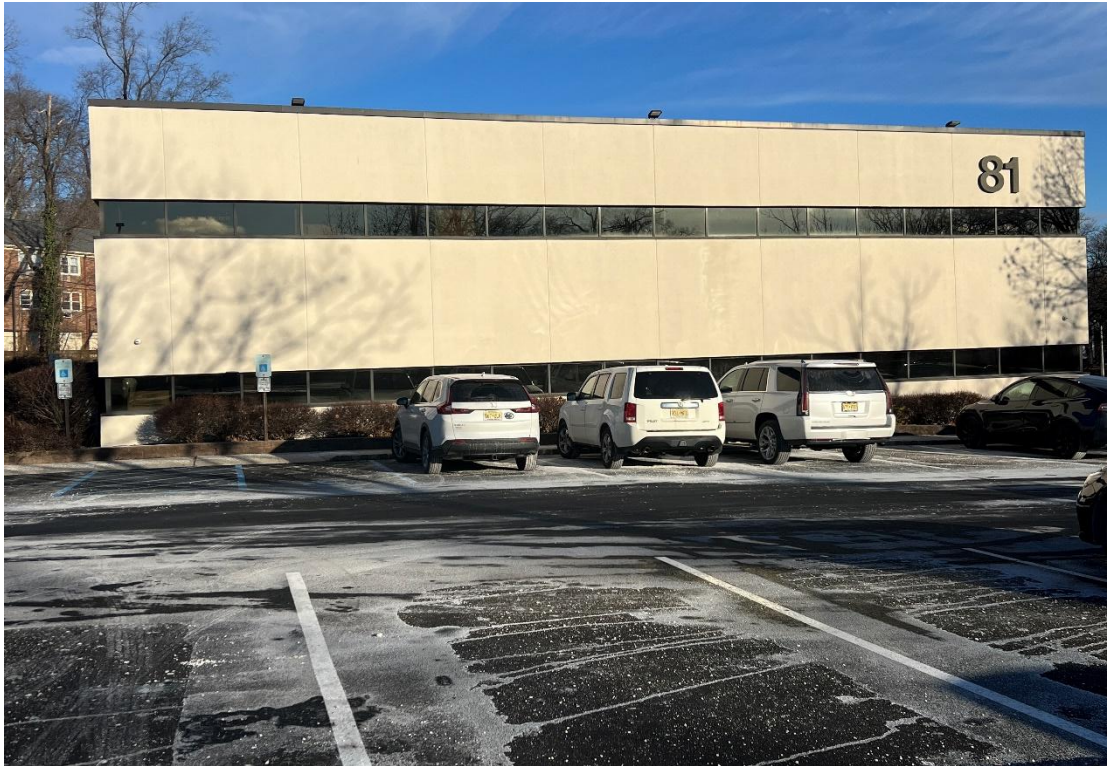
Figure 2: Front yard of 81 Northfield Ave from the southern side of the property (Northfield Ave)
