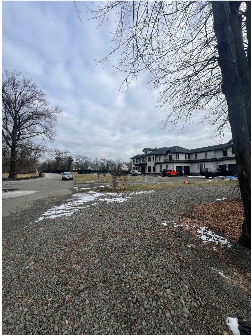
Figure 5: View of 40 Eagle Ridge Way from the site
