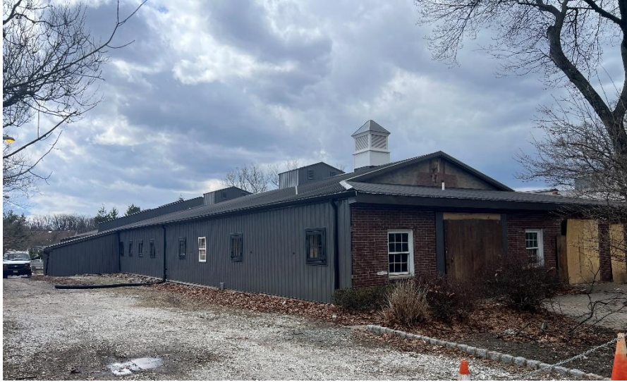
Figure 2: View of the site facing southwest from end of Eagle Ridge Way
