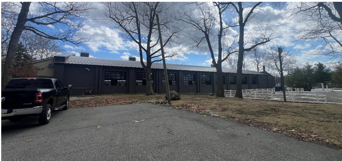
Figure 7: Existing parking lot area and side of the indoor riding arena
