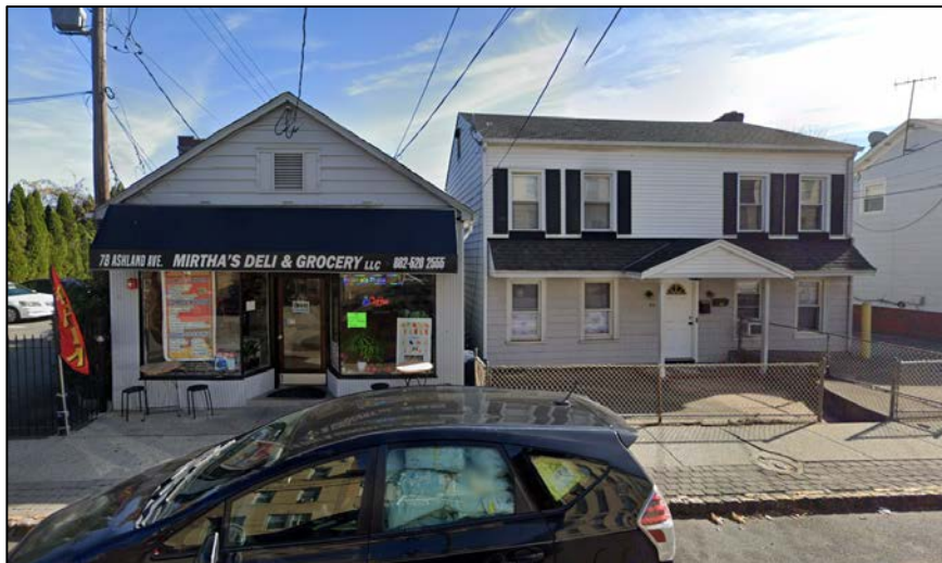
Photo 2: View of two of the four existing structures on the subject site. These building are located and 78 and 80 Ashland Avenue.
