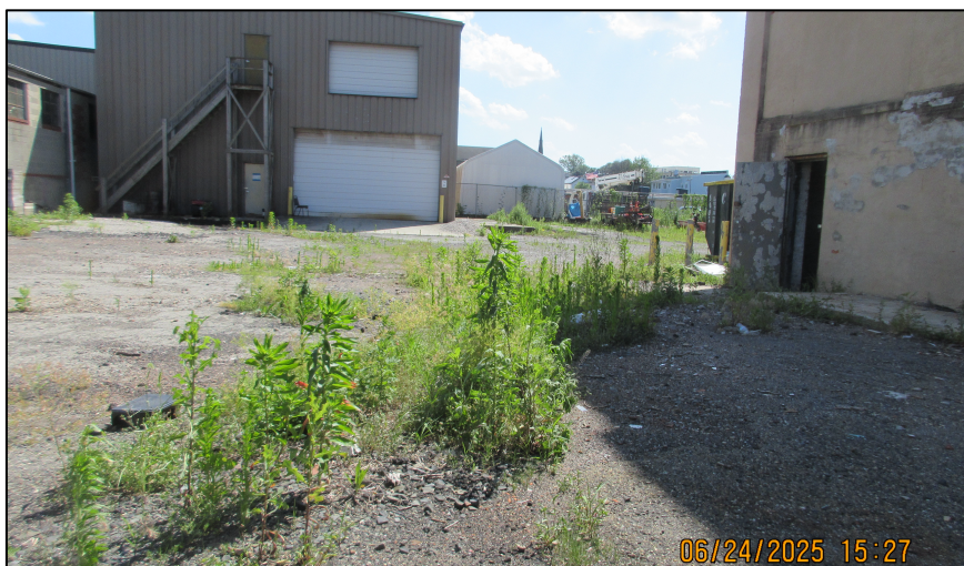
Photo 6: View looking south across the site towards the 2-story metal building. A row of parking stalls is proposed in the area in front of this building.
