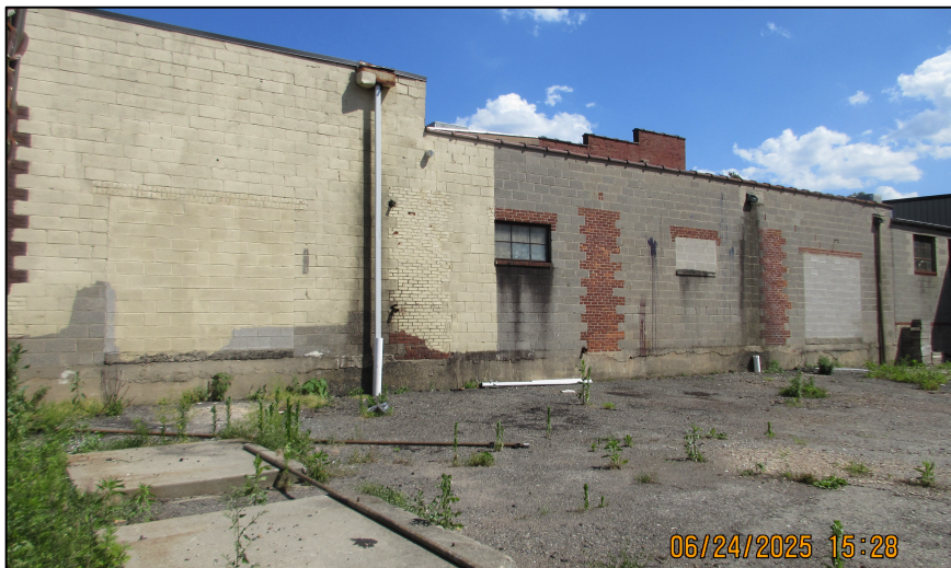
Photo 5: View showing the southern façade of the subject building.
