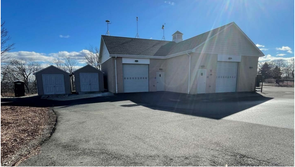
Front of existing building and driveway
