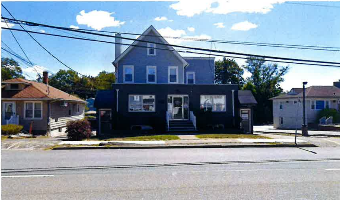
Figure 3 – View of the mixed-use building on Lot 11 (Source: njpropertyrecords.com)
