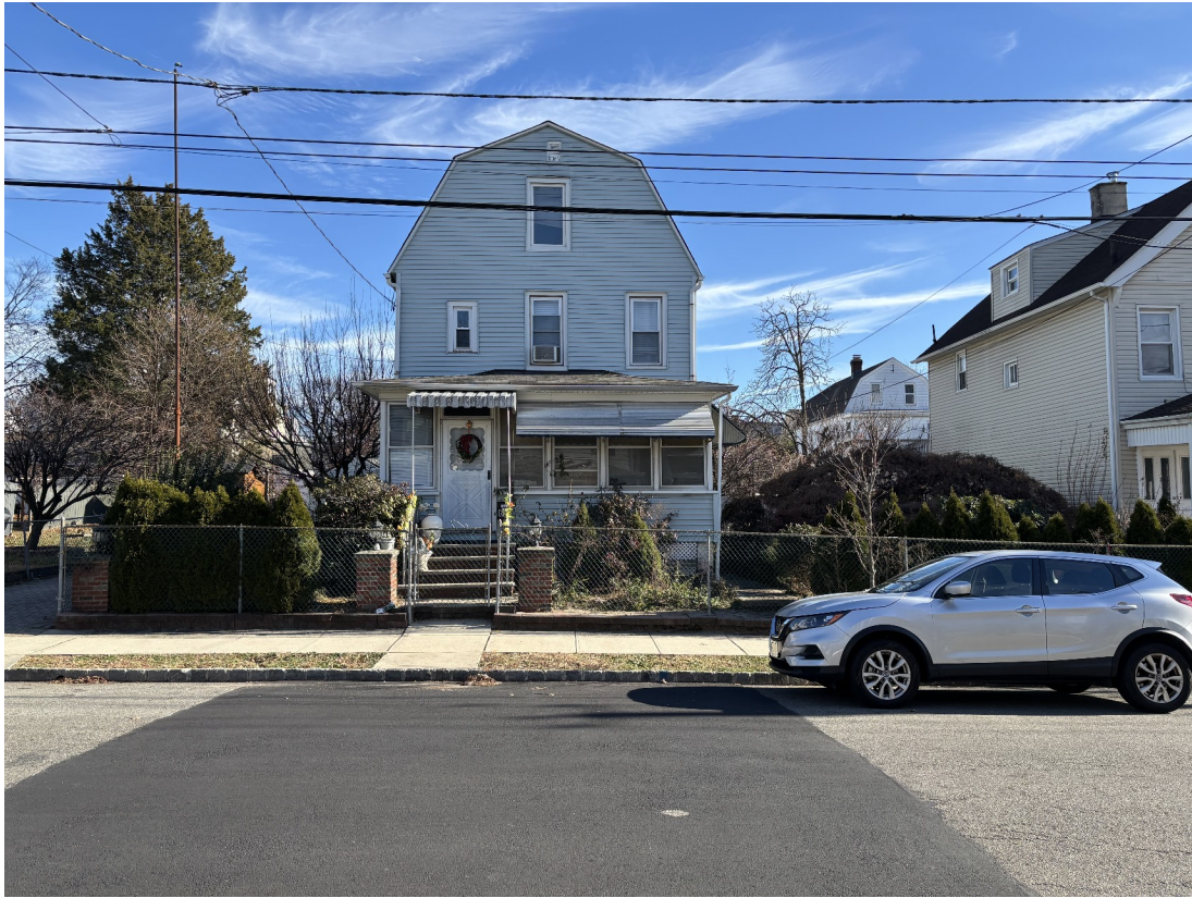
The above photo was taken by SE on 12/09/25 and depicts the front (westerly) facade of the existing building.
