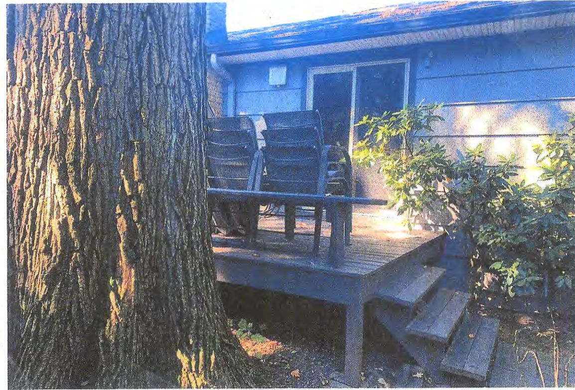
RIGHT SIDE OF DECK
