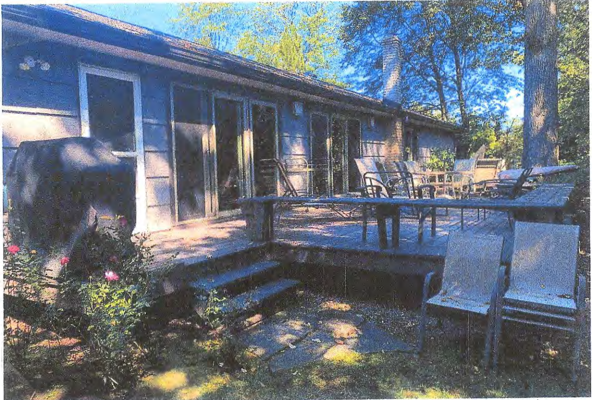
LEFT SIDE OF DECK
