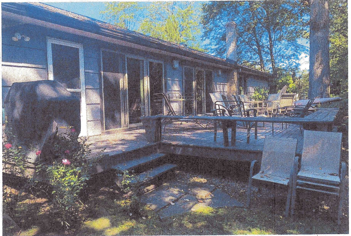
LEFT SIDE OF DECK
