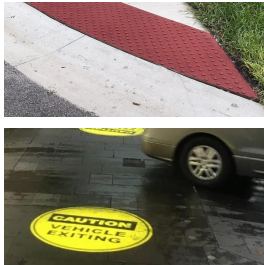
Detectable Warning: Textured Surface or Painted Sign
