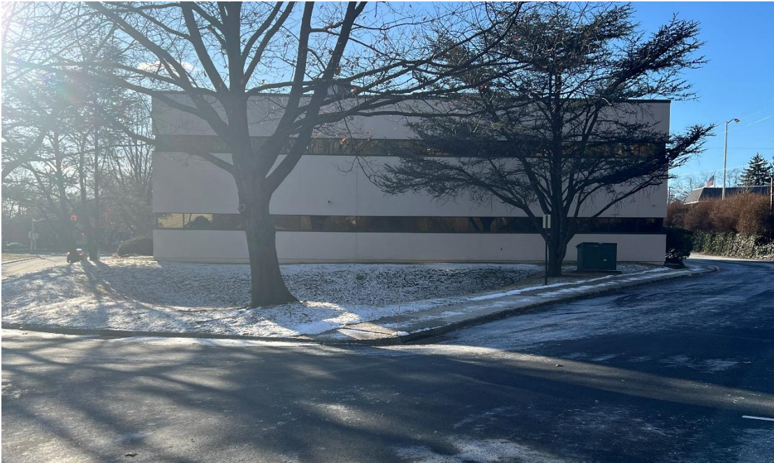
Figure 3: Rear of 81 Northfield Ave, looking south from rear parking lot area.
