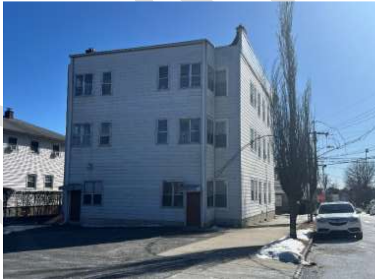
Figure 6: Rear of 61 Chestnut, a multi-family building located south of subject property at corner of Franklin Ave and Chestnut St.
