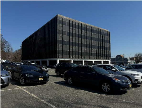
Figure 4: The office building viewed from the southern drive aisle
