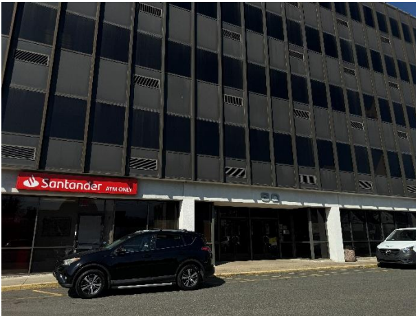
Figure 6: The office building's primary entrance
