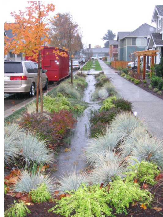
Bioswale example of stormwater best management practice
