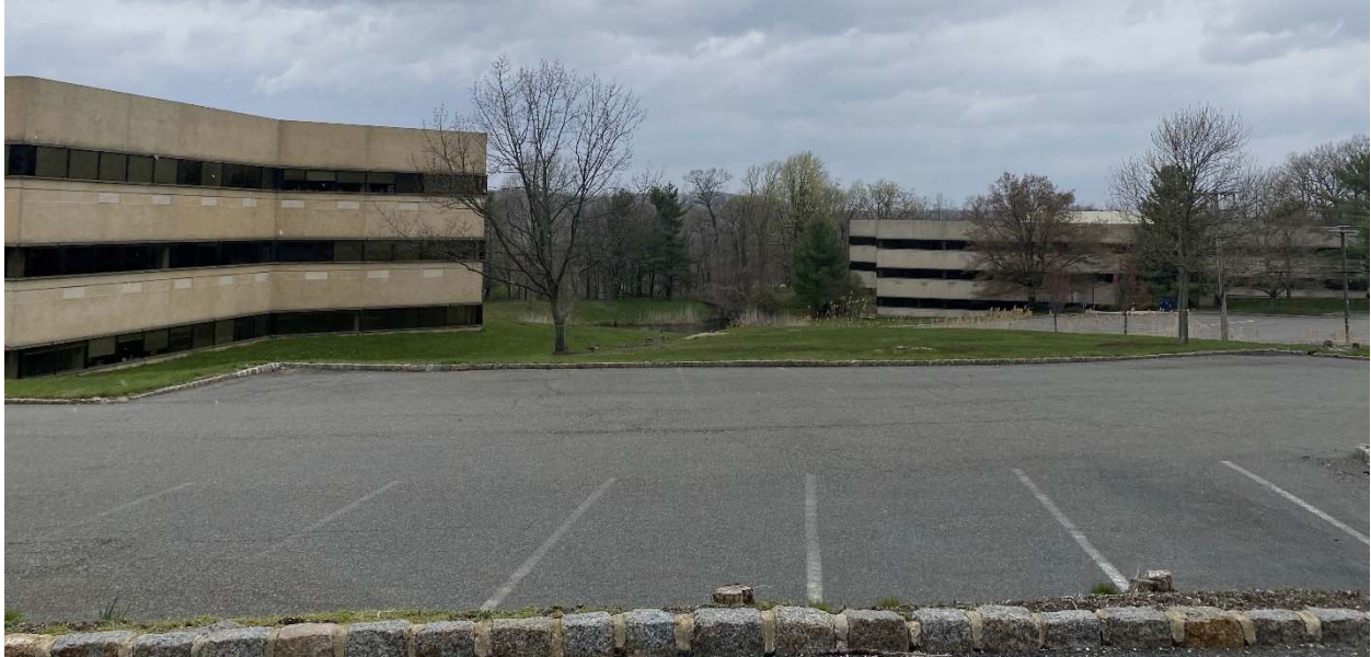
Existing office buildings to be removed and pond in between them
