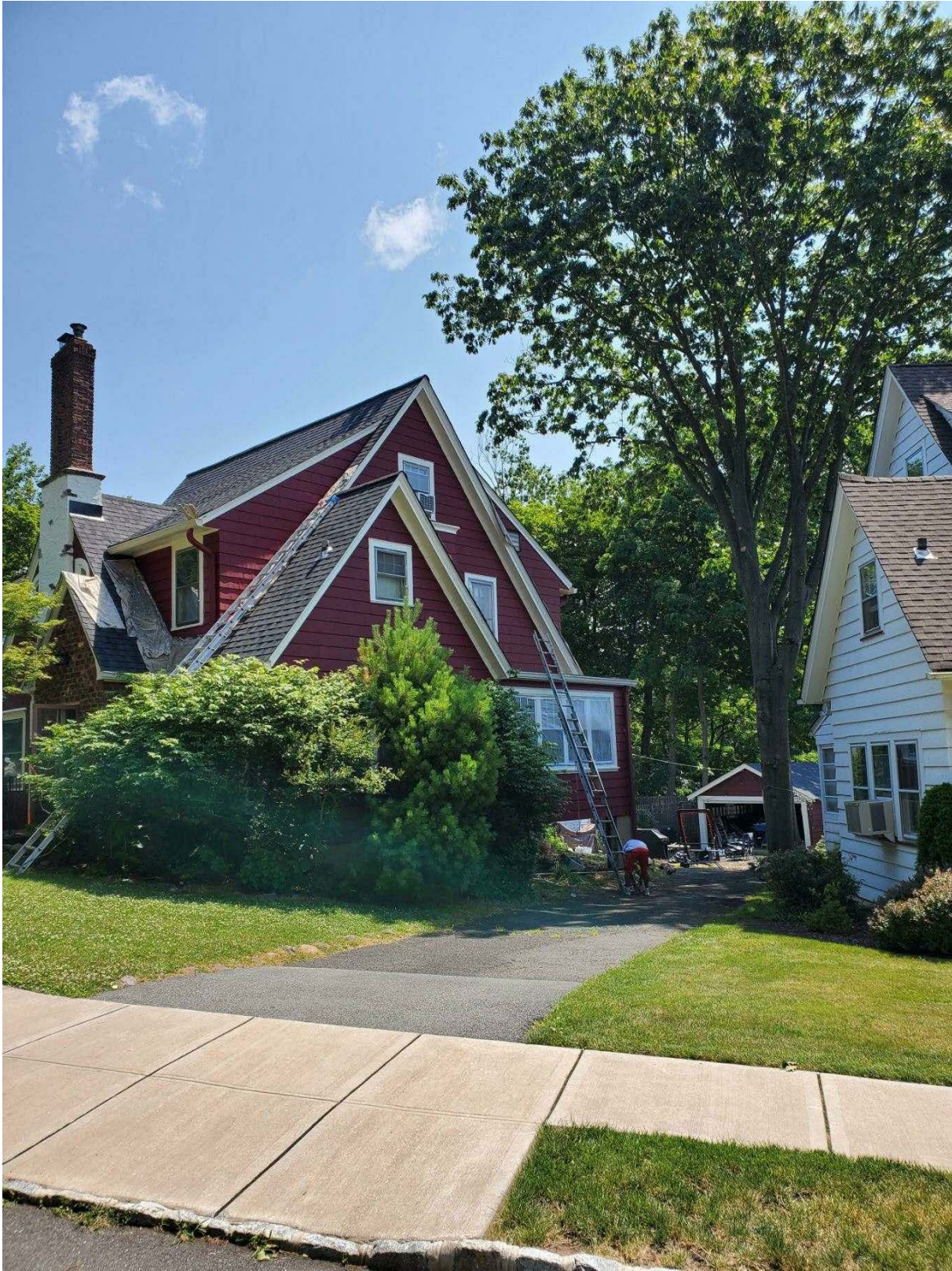
VIEW OF RIGHT SIDE OF HOUSE
