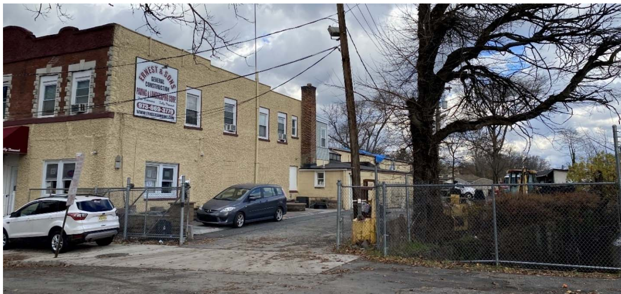
East driveway (provides access to rear of property)
