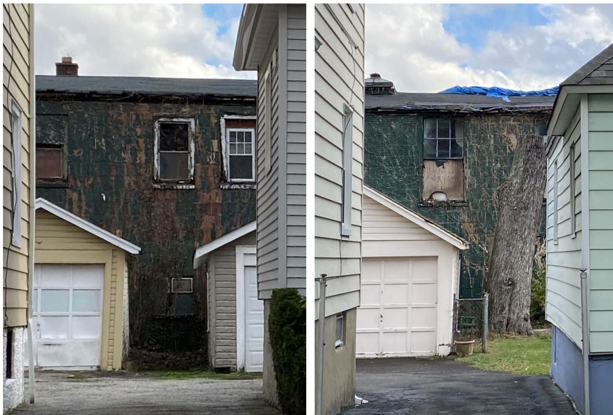
Two views of western wall of existing rear building from Central Place
