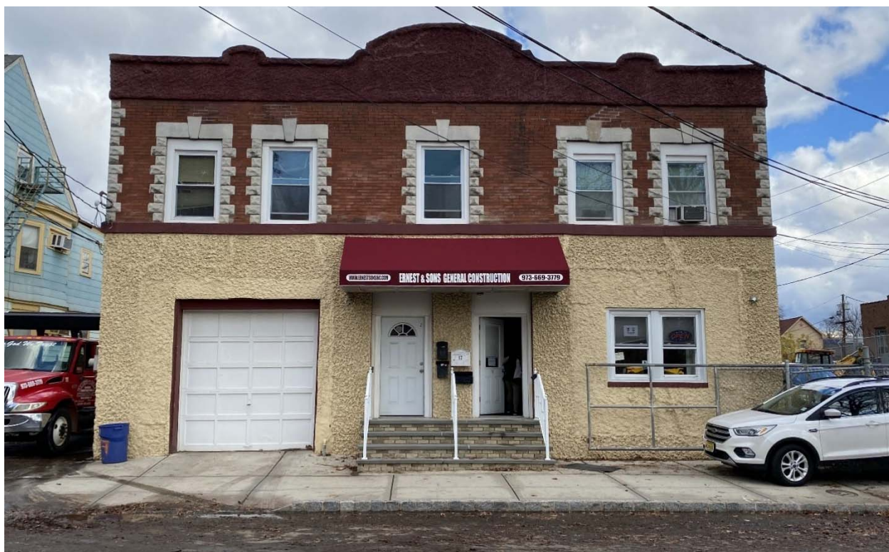
View of front building from Meeker Place
