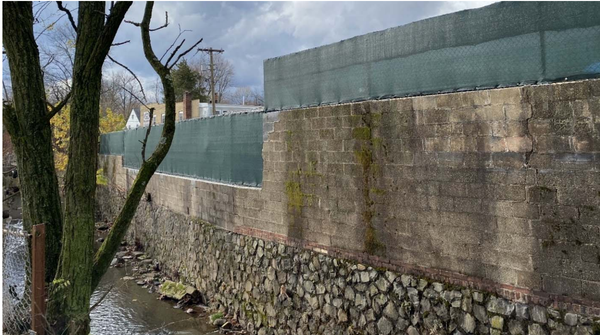
Improvements along eastern property line – looking southwest from Beach St. in Orange
