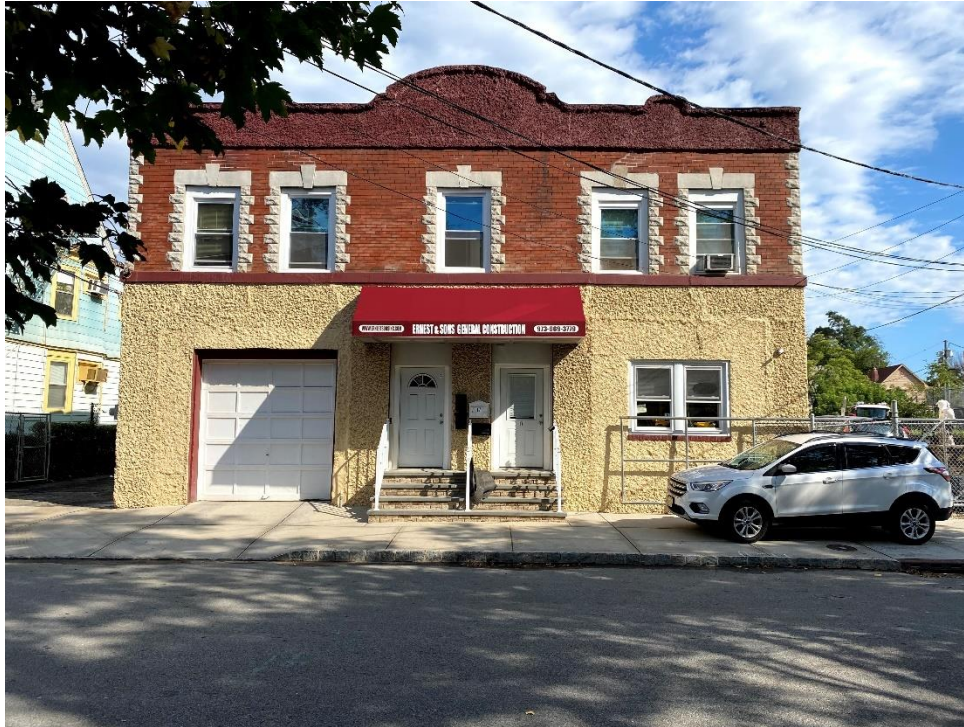
Figure 1: View of the mixed-use building on the subject property at 15 and 19 Meeker Street (Block 2, Lot 43.01 & 50), from Meeker Street viewing north.
