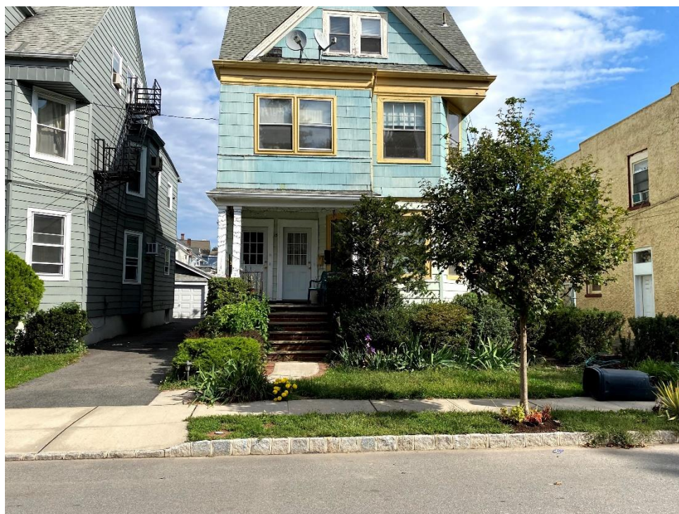
Figure 4: View of the property at 13 Meeker Street (Block 2, Lot 51) adjacent to the west of the subject property, from Meeker Street viewing north.
