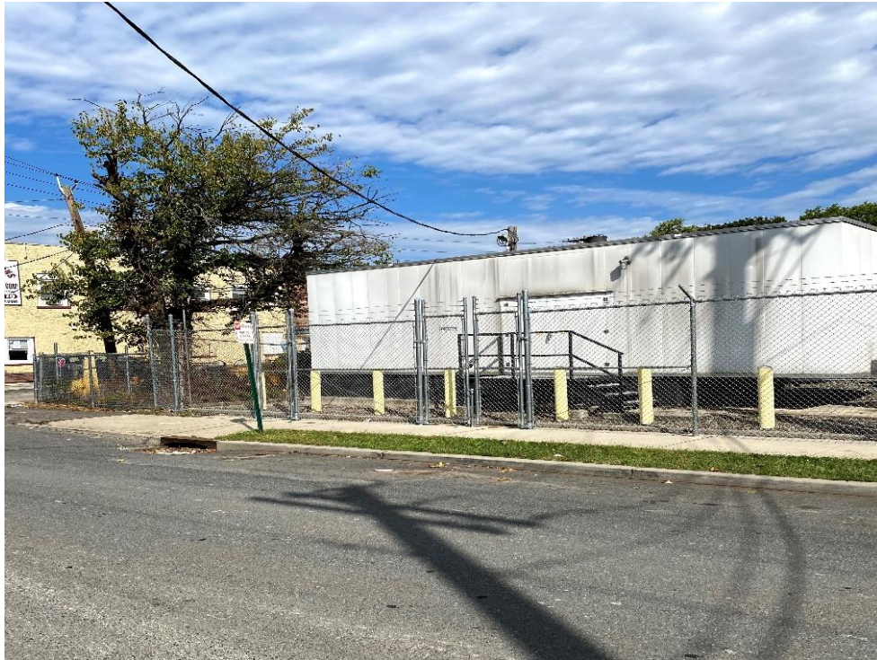
Figure 5: View of the property at 362 Chestnut Street (Block 6201, Lot 1) adjacent to the east of the subject property, in Orange, from Chestnut Street viewing north.
