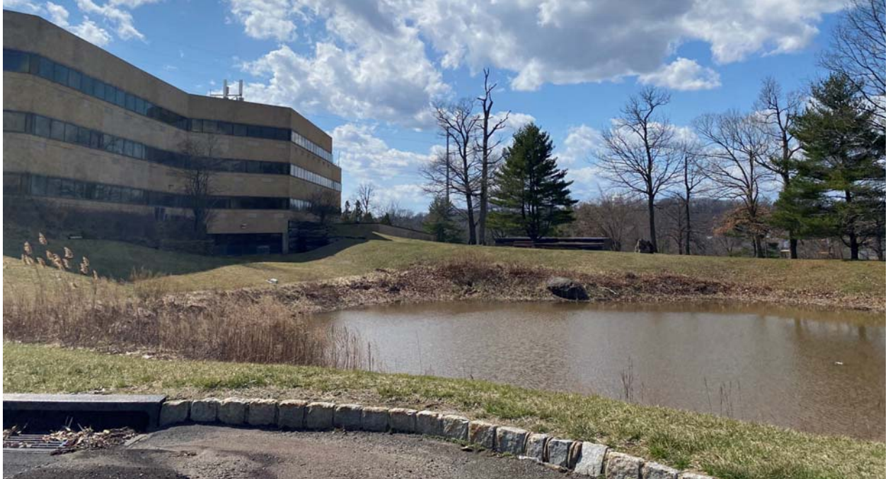
One of the existing office buildings to be removed and pond next to it
