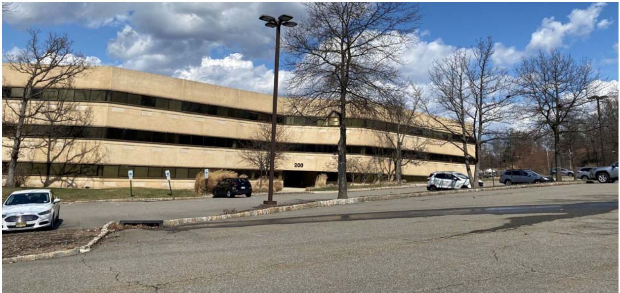
Looking northwest from existing parking lot towards 200 Executive Drive office building
