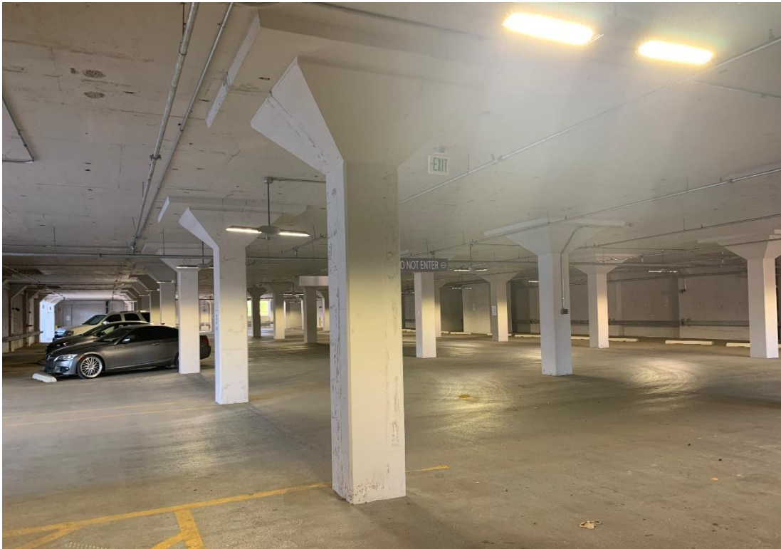
Photo 6: View of 3 rd floor of Harvard Printing I parking deck.
