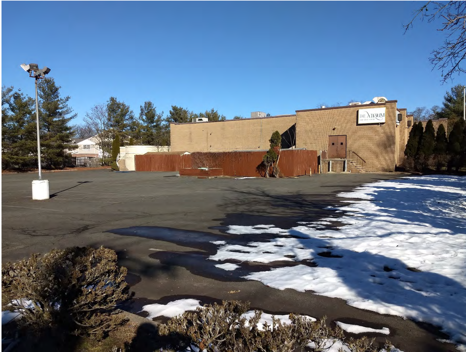
Site Photograph: View northeast from Eagle Rock Avenue west entrance of existing catering facility
