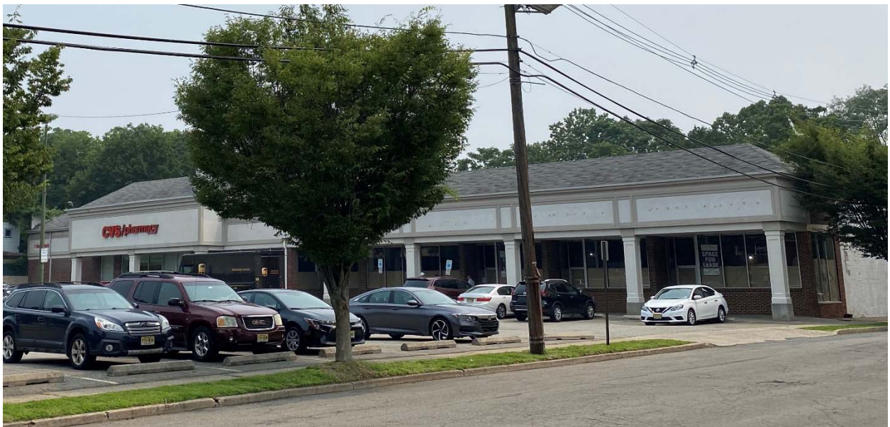
Views of portion of building where façade sign proposed
