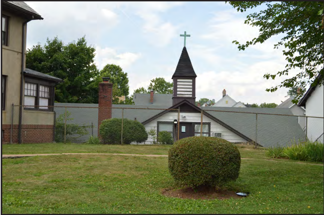
Photograph 28. View of the community center showing the side (southwest) elevation, view looking northeast (Photographer: Eryn Boyce, July 2019) [HRI Neg. #18039/D1:272].
