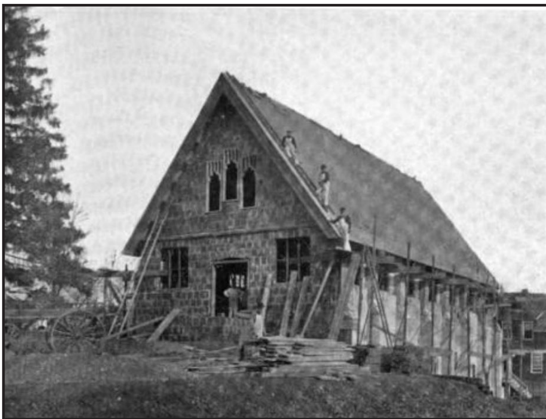
Photograph 29. Oblique view of Holy Trinity Episcopal Church under construction. Note the hollow structural clay tile load-bearing walls. 1907. Source: Schuyler 1909.
