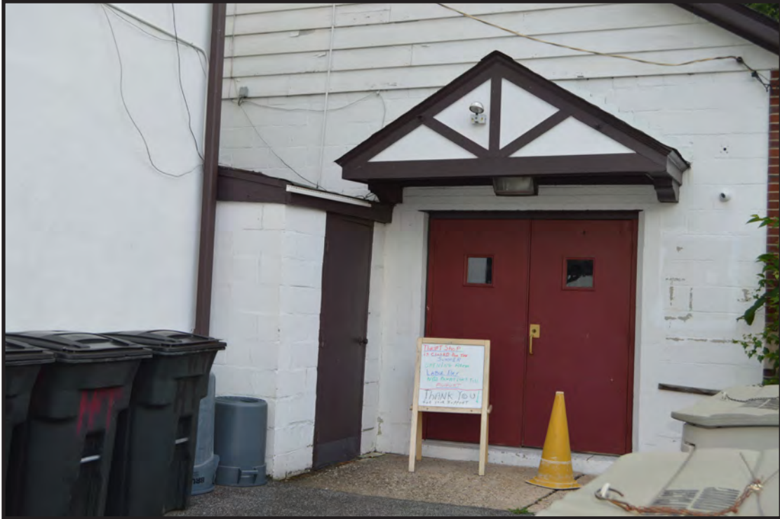
Photograph 9. View of the concrete-block passageway connecting the Holy Trinity Episcopal Church basement to the community center, view looking west (Photographer: Eryn Boyce, July 2019) [HRI Neg. #18039/D1: 268].
