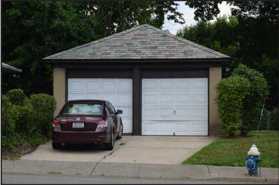
Photograph 26. View of the garage showing the front (southwest) elevation, view looking northeast (Photographer: Eryn Boyce, July 2019) [HRI Neg. #18039/D1:245].
