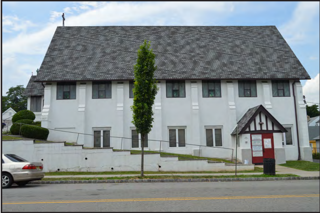
Photograph 3. View of Holy Trinity Episcopal Church showing the side (southeast) elevation, view looking northwest (Photographer: Eryn Boyce, July 2019) [HRI Neg. #18039/D1: 206].
