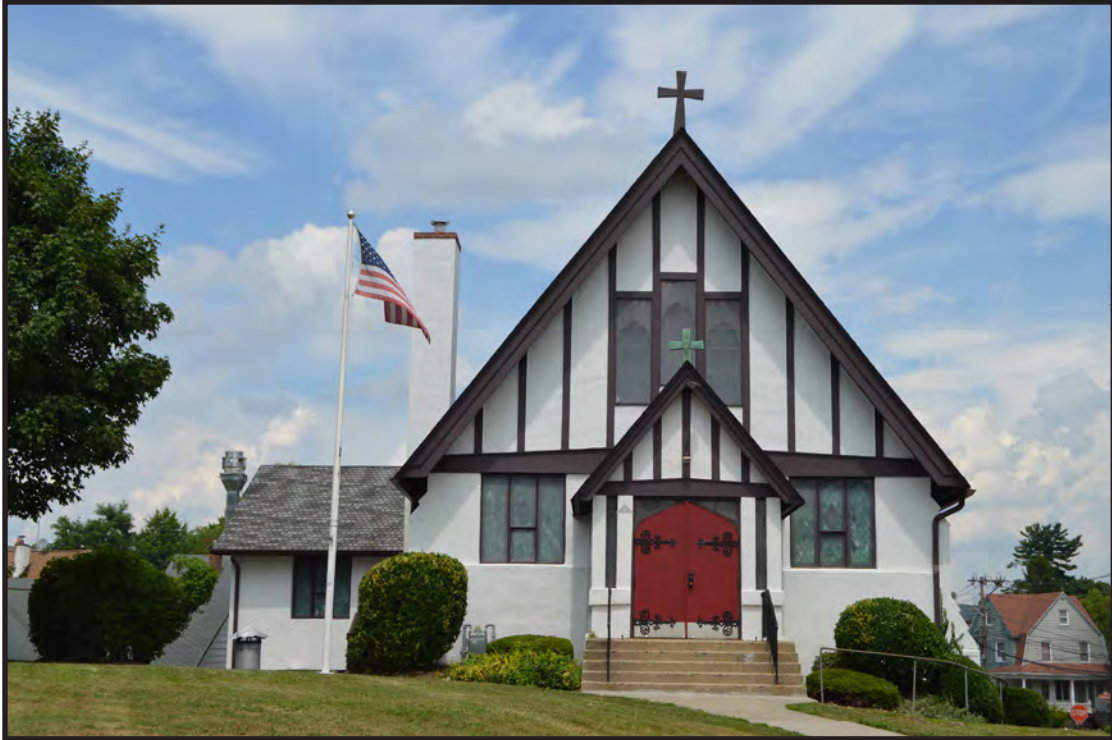
Photograph 1. View of Holy Trinity Episcopal Church showing the front (southwest) elevation, view looking northeast (Photographer: Eryn Boyce, July 2019) [HRI Neg. #18039/D1:196].
