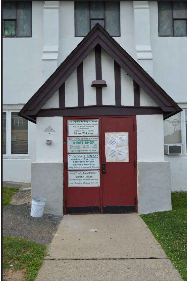
Photograph 8. View of basement entry, view looking northwest (Photographer: Eryn Boyce, July 2019) [HRI Neg. #18039/D1: 298].
