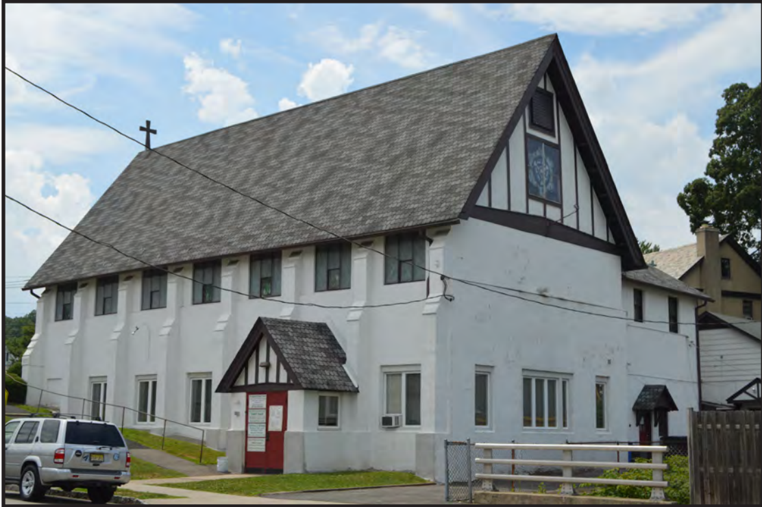
Photograph 7. Oblique view of Holy Trinity Episcopal Church showing the side (southeast) and rear (northwest) elevations, view looking west (Photographer: Eryn Boyce, July 2019) [HRI Neg. #18039/D1: 210].
