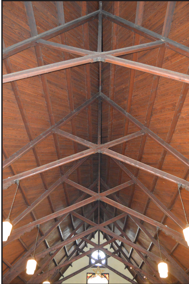
Photograph 13. View of the interior of Holy Trinity Episcopal Church showing the exposed roof framing, view looking northwest towards the choir and altar (Photographer: Eryn Boyce, July 2019) [HRI Neg. #18039/D1: 121].
