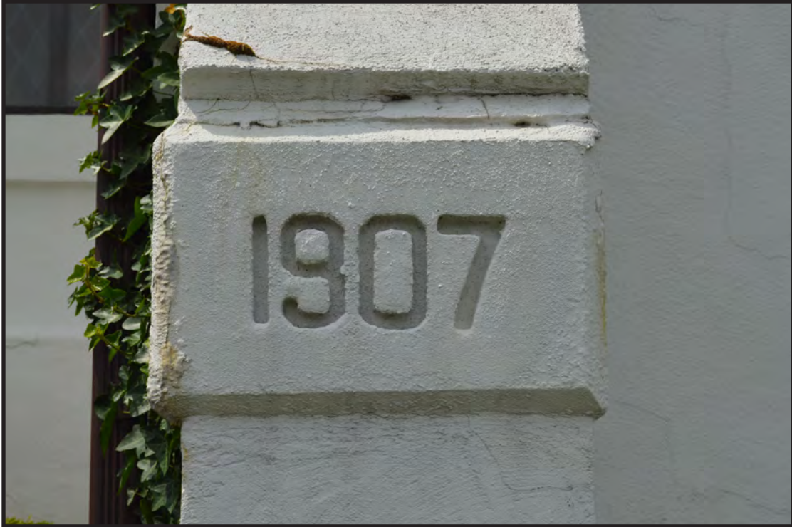
Photograph 5. View Holy Trinity Episcopal Church date stone, view looking northwest (Photographer: Eryn Boyce, July 2019) [HRI Neg. #18039/D1: 203].
