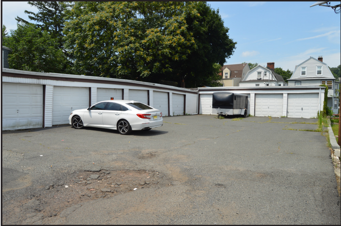
Photograph 14. View of the circa 1930 garage located behind the State Diner, view looking west (Photographer: Eryn Boyce, July 2019) [HRI Neg. #18039/D1:071].
