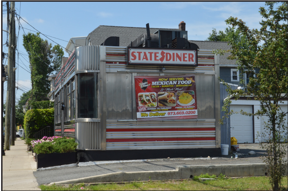
Photograph 4. View of the side (north) elevation of the State Diner, view looking southeast (Photographer: Eryn Boyce, July 2019) [HRI Neg. #18039/D1: 001].
