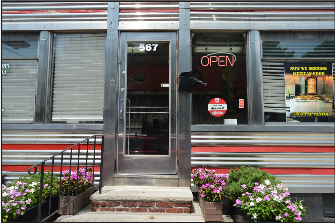
Photograph 7. Detail of the front entry to the State Diner, view looking northwest (Photographer: Eryn Boyce, July 2019) [HRI Neg. #18039/D1: 074].
