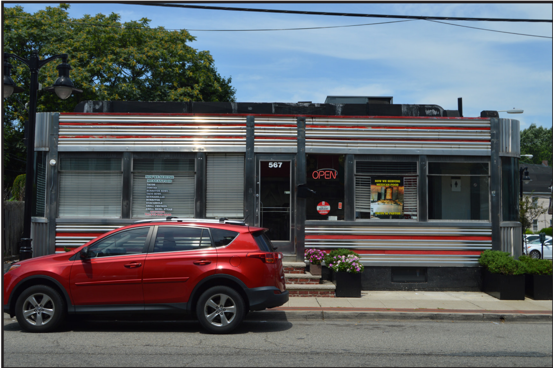
Photograph 2. View of the front (east) elevation of the State Diner, view looking northwest (Photographer: Eryn Boyce, July 2019) [HRI Neg. #18039/D1: 059].
