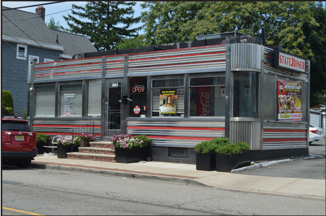
Photograph 1. Oblique view of the State Diner showing the front (east) and side (north) elevations, view looking southwest (Photographer: Eryn Boyce, July 2019) [HRI Neg. #18039/D1:057].
