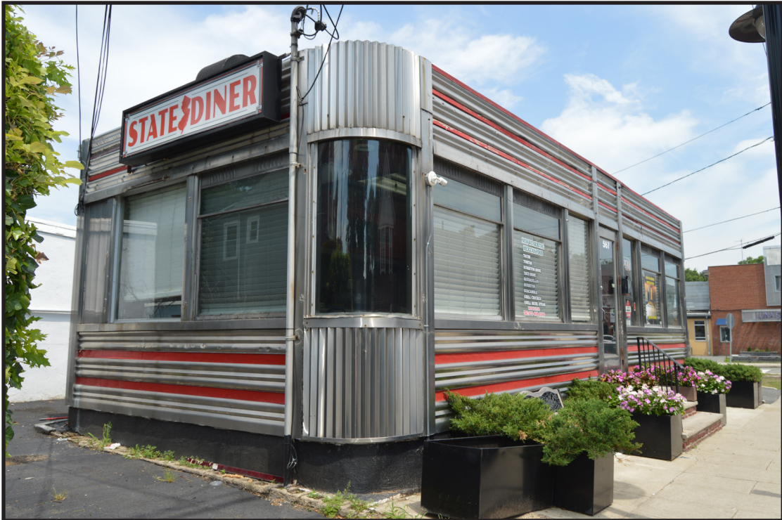
Photograph 3. Oblique view of the State Diner showing the front (east) and side (south) elevations, view looking north (Photographer: Eryn Boyce, July 2019) [HRI Neg. #18039/D1: 064].
