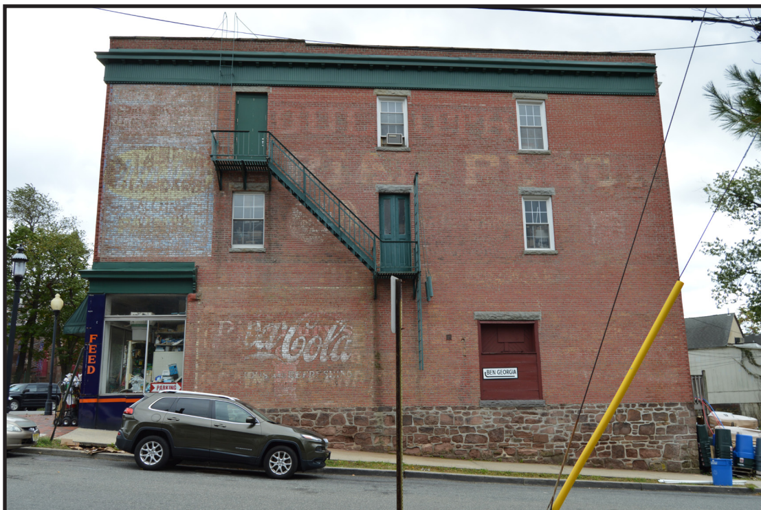
Photograph 5. View of the Hedges Block showing the side (north) elevation, view looking southeast (Photographer: Eryn Boyce, October 2019) [HRI Neg. #19016/D1: 082].
