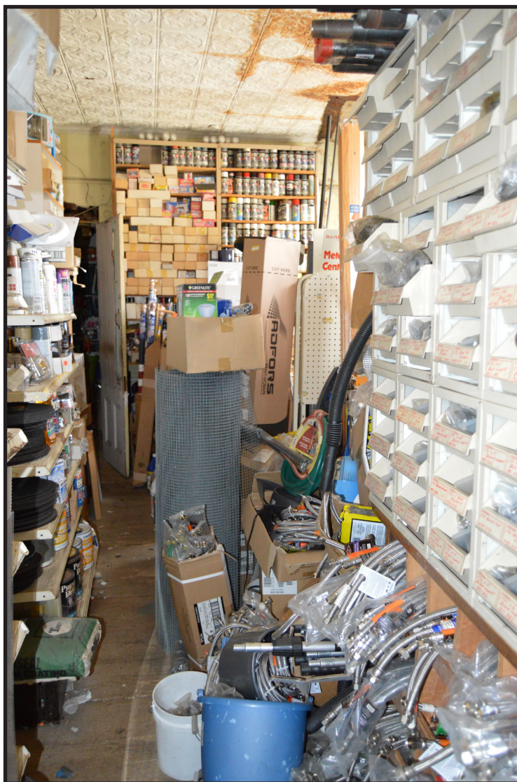
Photograph 21. View of the interior of the Hedges Block showing the northern half of the second floor and its wood plank floors, view looking southeast. Note the original pressed-tin ceiling (Photographer: Eryn Boyce, October 2019) [HRI Neg. #19106/D1:022].
