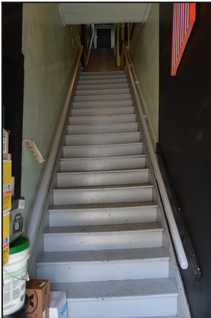
Photograph 7. View of interior of the Hedges Block showing the central staircase to the second and third floors, view looking southwest (Photographer: Eryn Boyce, October 2019) [HRI Neg. #19016/D1: 016].
