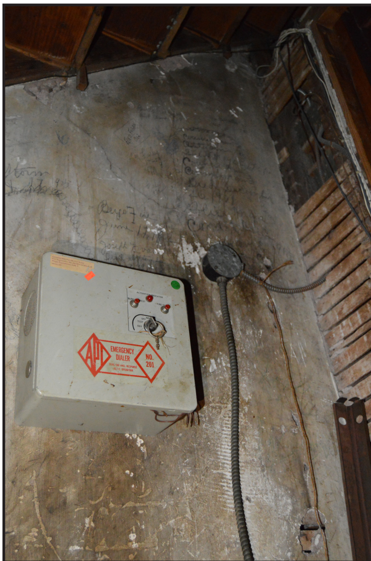
Photograph 16. View of the basement beneath Main St. Liquors showing the handwritten notes on the plaster walls, view looking southwest (Photographer: Eryn Boyce, October 2019) [HRI Neg. #18039/D1:071].
