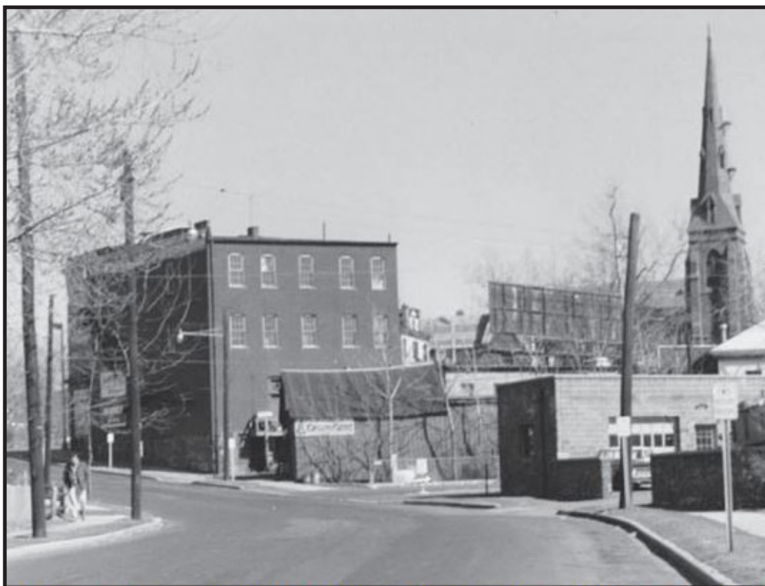
Photograph 31. Oblique view of the Hedges Block showing the wood-frame storage sheds behind the building. No date. Source: Fagan 2016.
