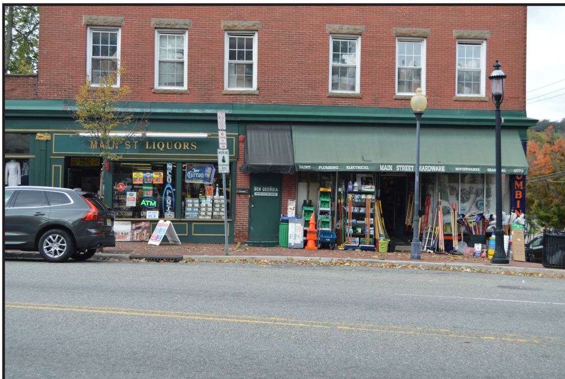
Photograph 4. View of the first-story storefronts at the Hedges Block, view looking southwest (Photographer: Eryn Boyce, October 2019) [HRI Neg. #19016/D1: 087].
