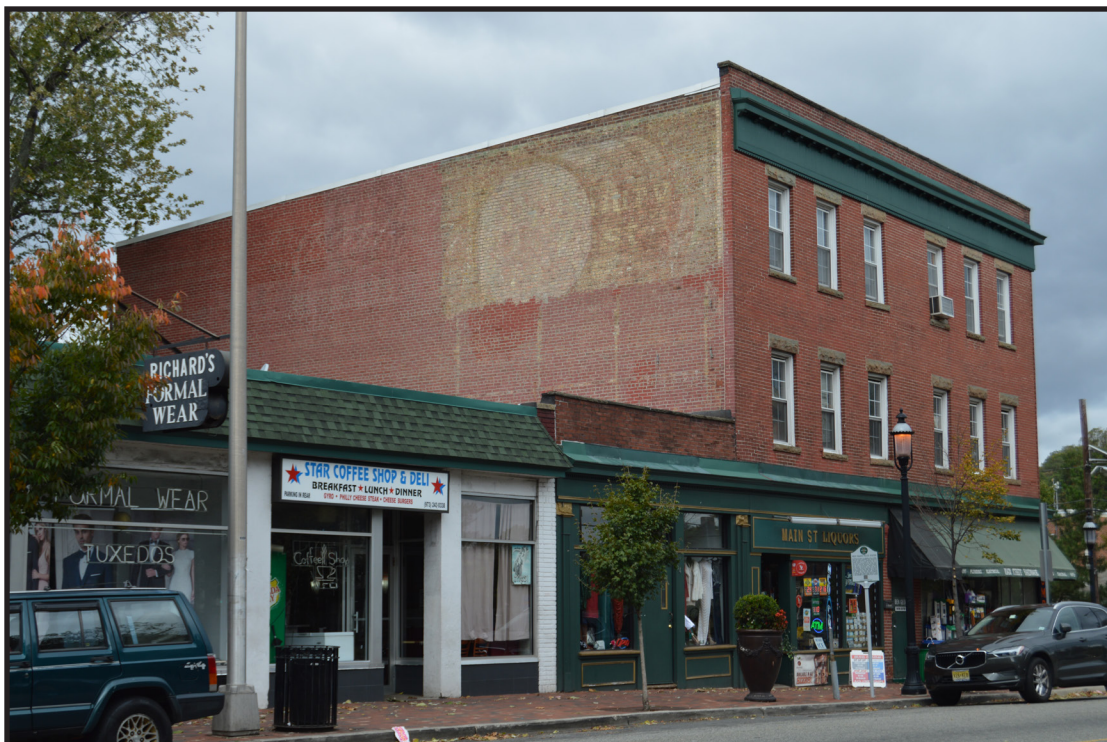
Photograph 32. View of 52 and 54 Main Street, view looking northwest (Photographer: Eryn Boyce, October 2019) [HRI Neg. #19016/D1:86].
