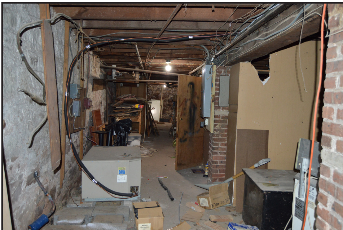
Photograph 14. View of the basement beneath Main St. Liquors, view looking northeast (Photographer: Eryn Boyce, October 2019) [HRI Neg. #19016/D1:076].
