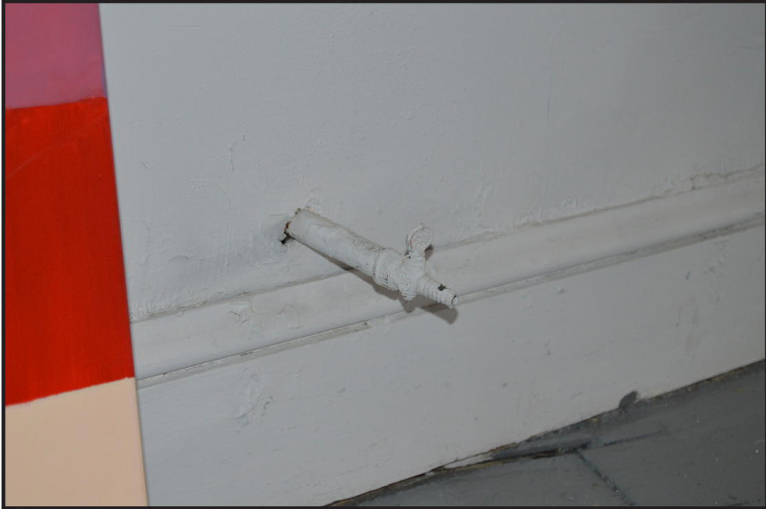
Photograph 28. Detail of one of the sewing machine hookups located in the southern half of the third floor, view looking northeast (Photographer: Eryn Boyce, October 2019) [HRI Neg. #19016/D1:061].
