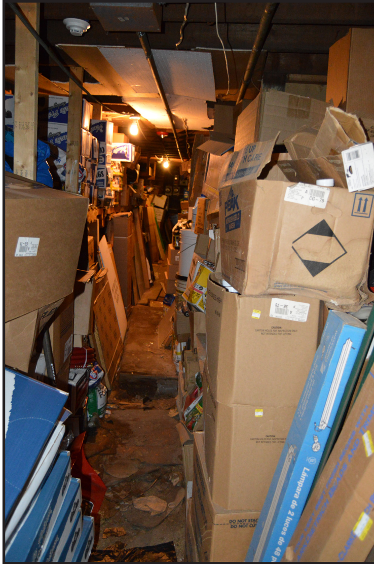
Photograph 11. View of the basement beneath Main Street Hardware, view looking northeast (Photographer: Eryn Boyce, October 2019) [HRI Neg. #19016/D1: 010].
