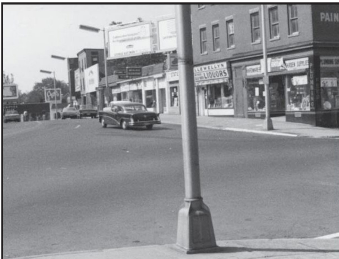
Photograph 29. View of Main Street showing the first-story storefront of the Hedges Block (right). 1960s. Source: Fagan 2016.
