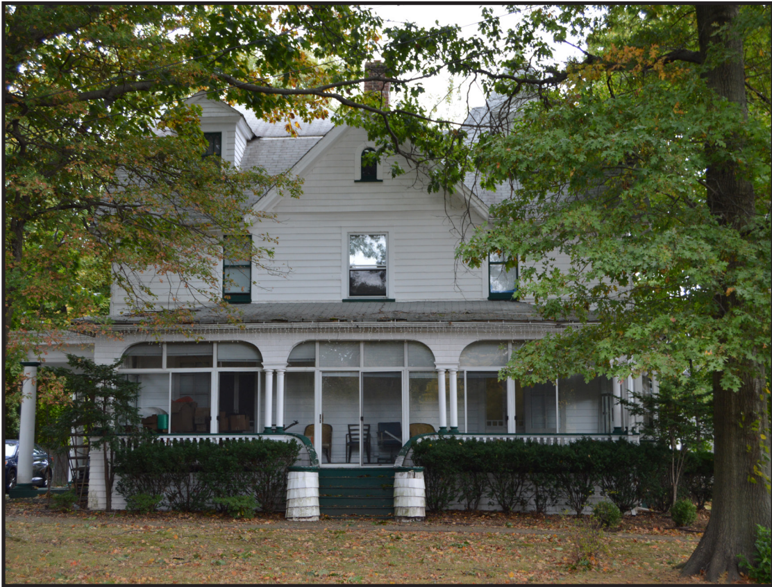
Photograph 3. View of the Williams/McManus/Lehmann House showing the side (south) elevation, view looking northeast (Photographer: Eryn Boyce, October 2019) [HRI Neg. #19016/D1: 091].
