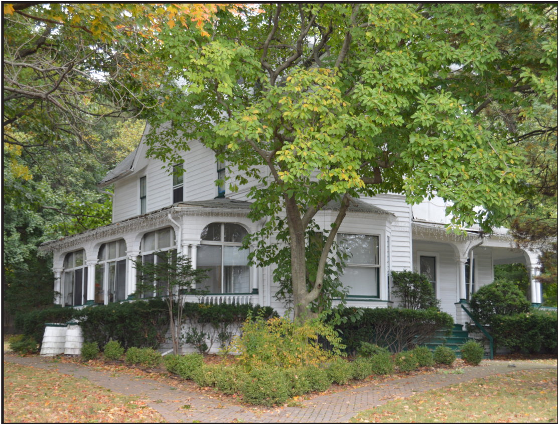
Photograph 2. Oblique view of the Williams/McManus/Lehmann House showing the front (east) and side (south) elevations, view looking northwest (Photographer: Eryn Boyce, October 2019) [HRI Neg. #19016/D1: 089].
