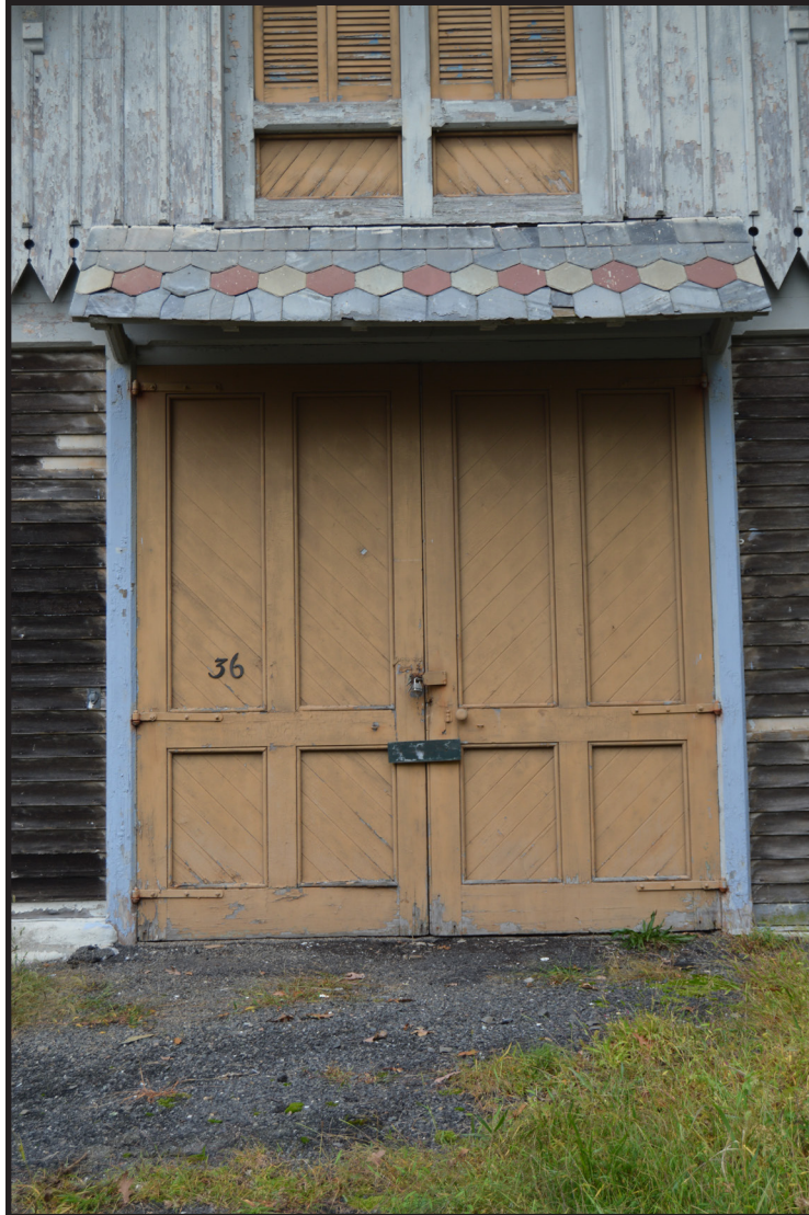
Photograph 9. View of shed-roof hood above carriage doors on the front (west) elevation, view looking southwest. Note the original pattern slate shingles (Photographer: Eryn Boyce, September 2020) [HRI Neg. #20054/D1:030].
