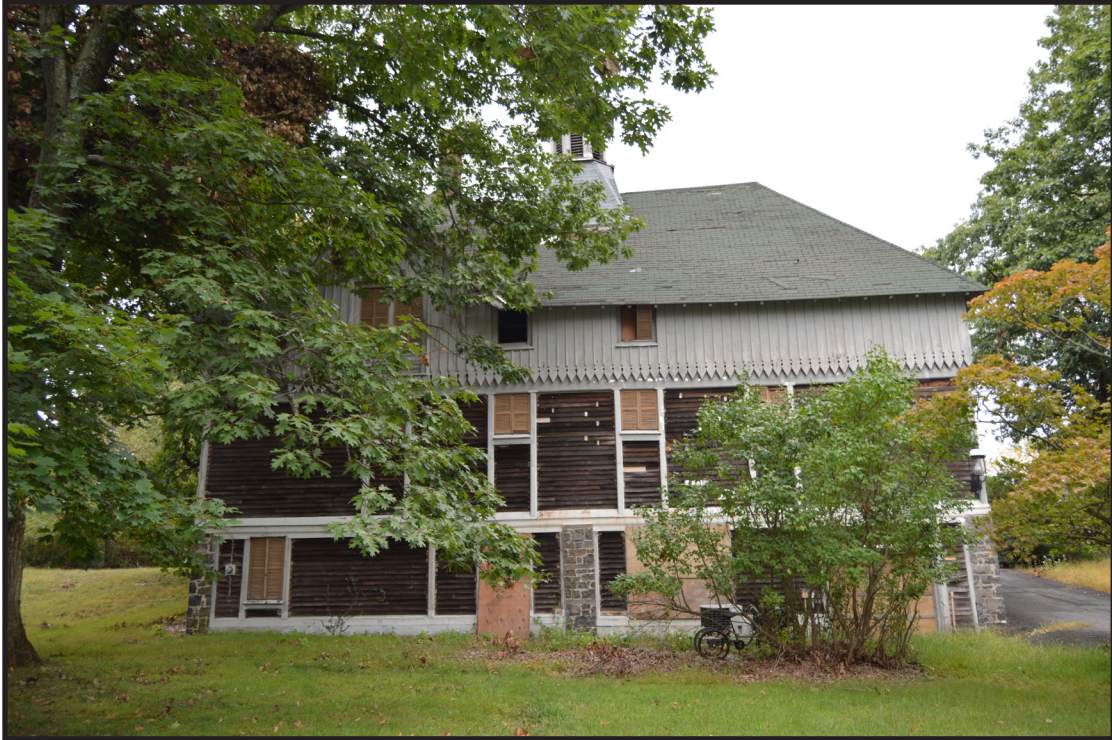
Photograph 5. View of George V. Hecker Carriage House showing the rear (east) elevation, view looking northeast (Photographer: Eryn Boyce, September 2020) [HRI Neg. #20054/D1:036].
