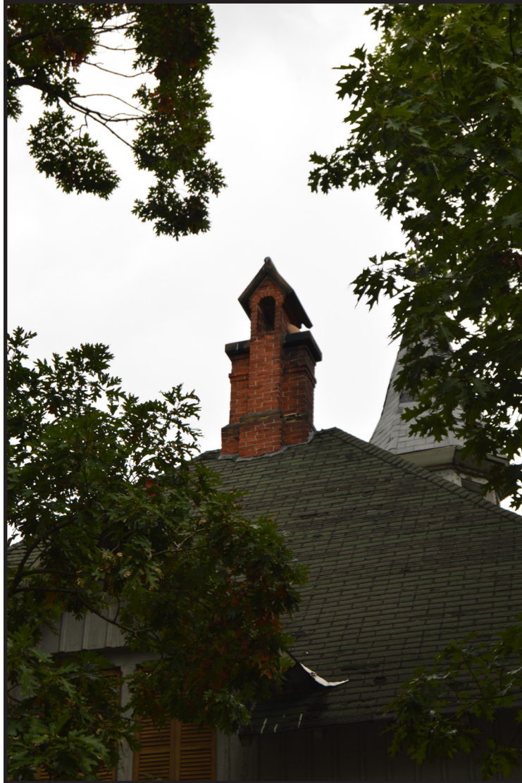
Photograph 3. View of George V. Hecker Carriage House chimney, view looking northeast (Photographer: Eryn Boyce, September 2020) [HRI Neg. #20054/D1:040].
