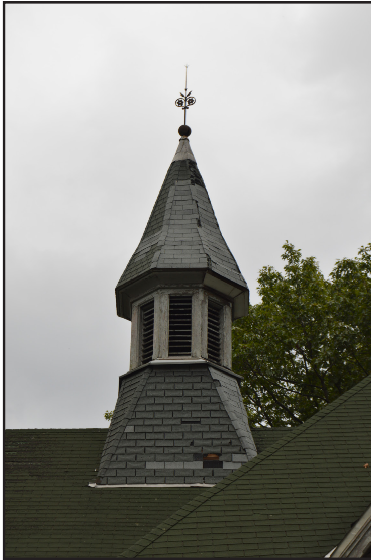
Photograph 2. View of George V. Hecker Carriage House ventilator, view looking southeast (Photographer: Eryn Boyce, September 2020) [HRI Neg. #20054/D1:048].
