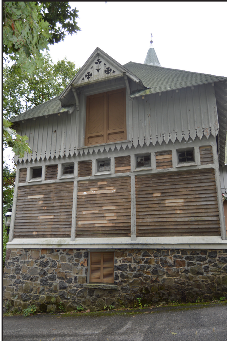
Photograph 6. View of George V. Hecker Carriage House showing the side (north) elevation, view looking southwest (Photographer: Eryn Boyce, September 2020) [HRI Neg. #20054/D1:035].
