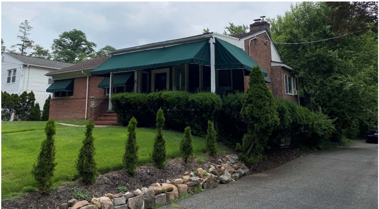
View of southern property line from front
