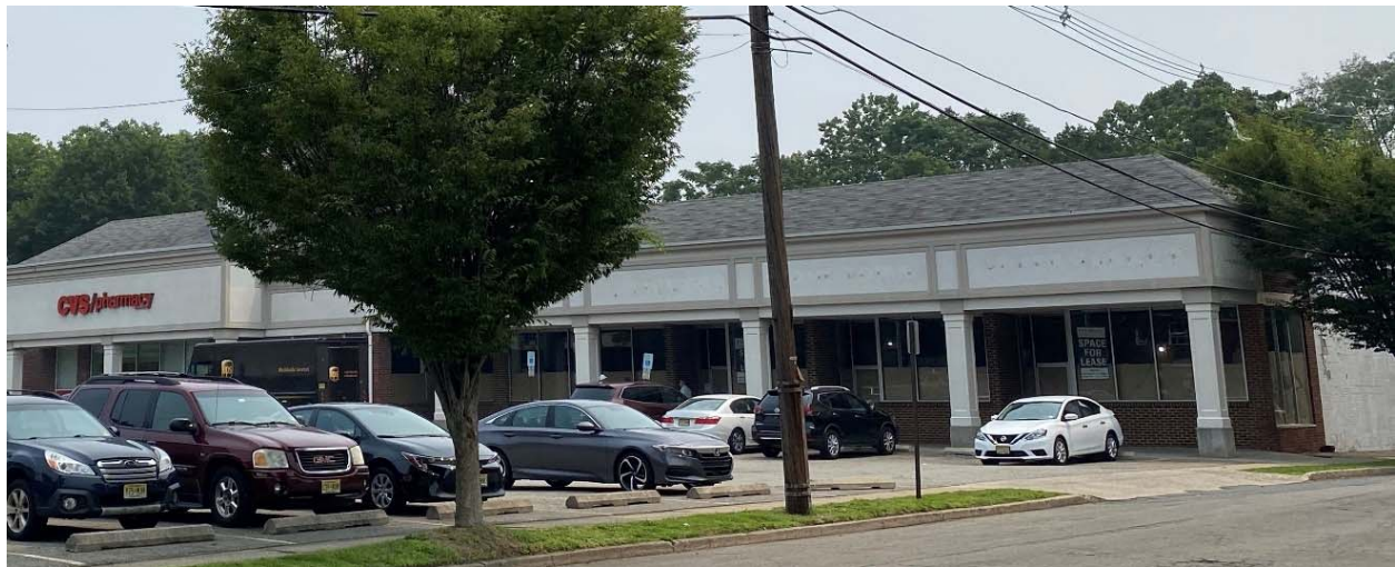
Views of portion of building where illuminated façade sign is proposed
