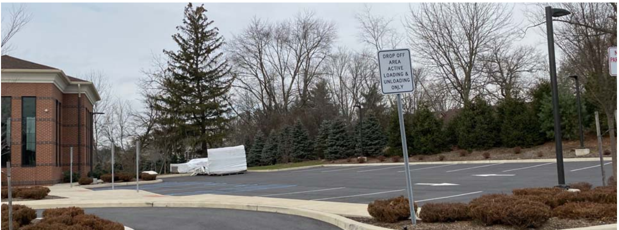
Existing parking lot and buffering on side property line
