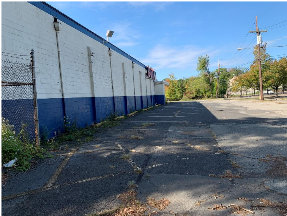
Figure 4: View of the north side of the project site, viewing southwest.
