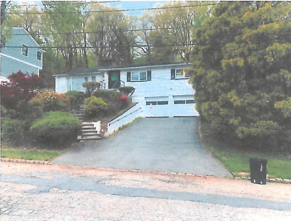
Photo 4 House immediately to the North on Cleveland. Note railing on wall coming down from the garage.
