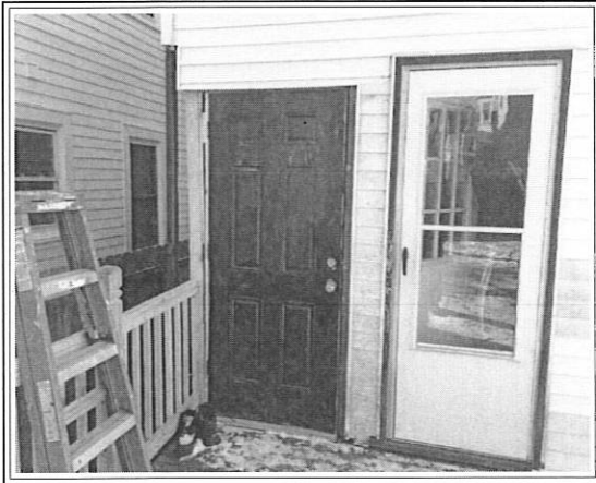
Rear siding repaired.
