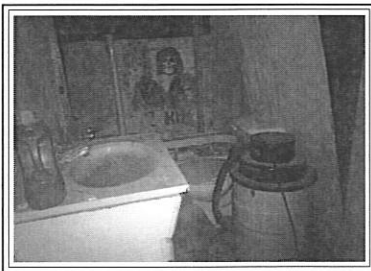
Basement Bath (non functional)
