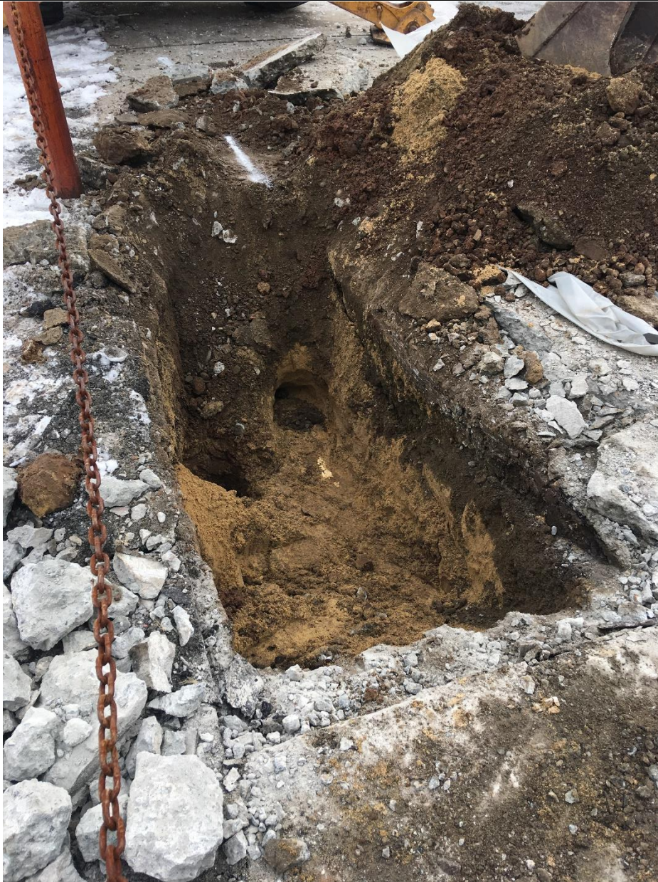
PHOTO 3: Looking east at north side of test pit located in the sidewalk along Eagle Rock Avenue (January 19, 2018).
