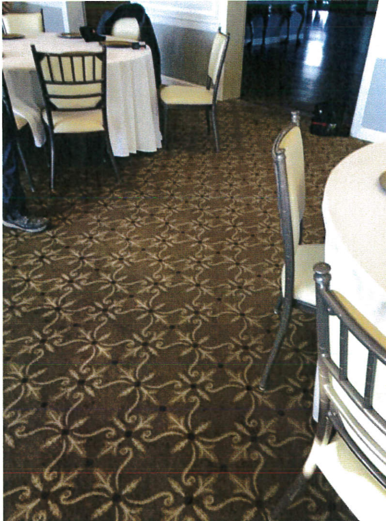
105 105-Pre-Mitigation - Dining Room Date Taken: 12/26/2022 (Zone 1) 2
