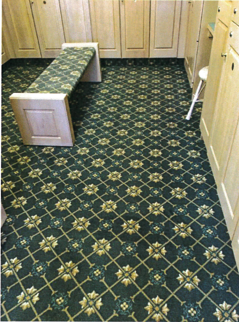
150 150-Pre-Mitigation - Locker room Date Taken: 12/26/2022 (Zone 1) 4
