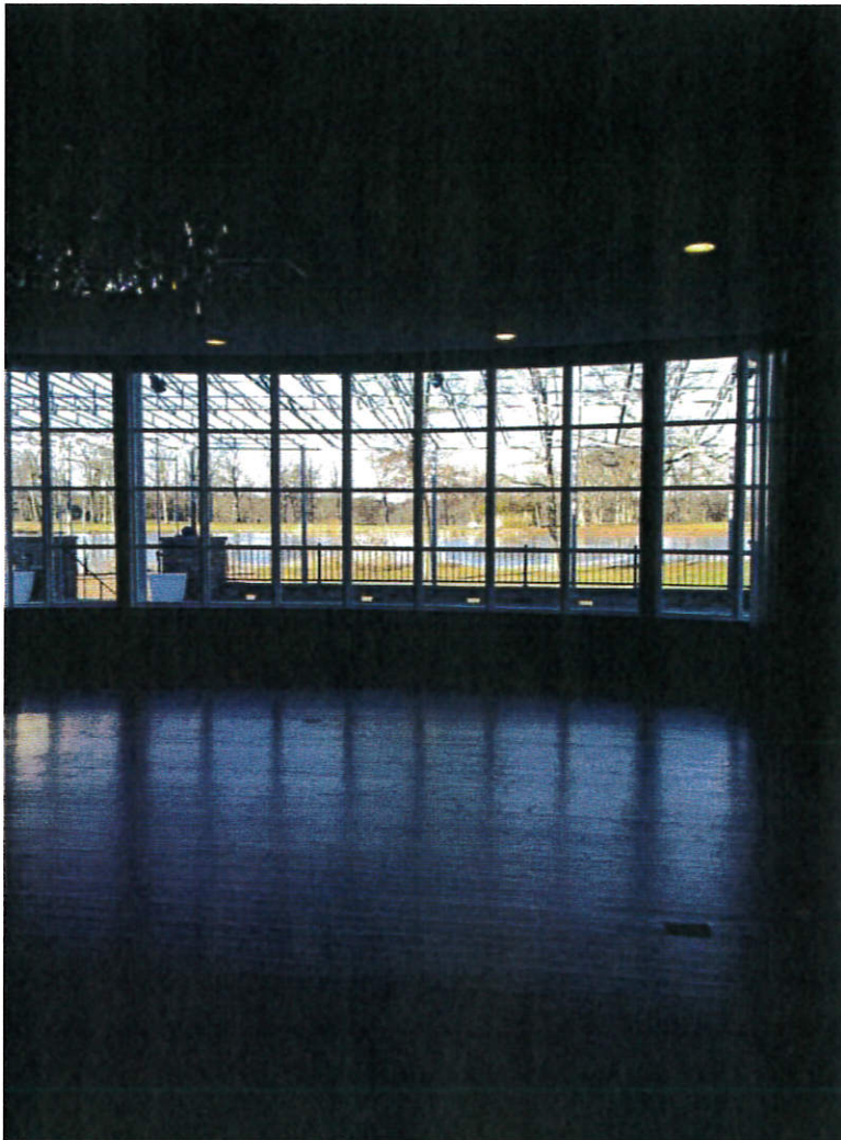
98 98-Pre-Mitigation - Ball room Date Taken: 12/26/2022 (Zone 2) 8
