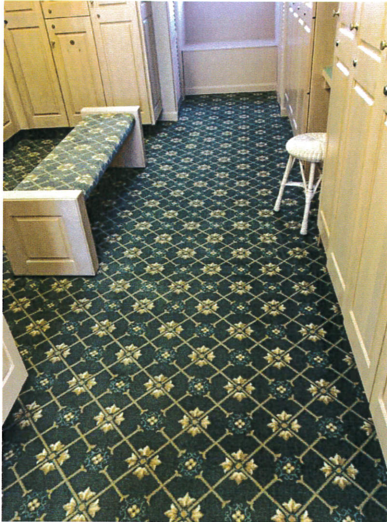
152 152-Pre-Mitigation - Locker room Date Taken: 12/26/2022 (Zone 1) 6
