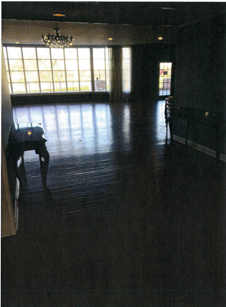
118 118-Pre-Mitigation - Foyer (Zone 2) Date Taken: 12/26/2022 14
