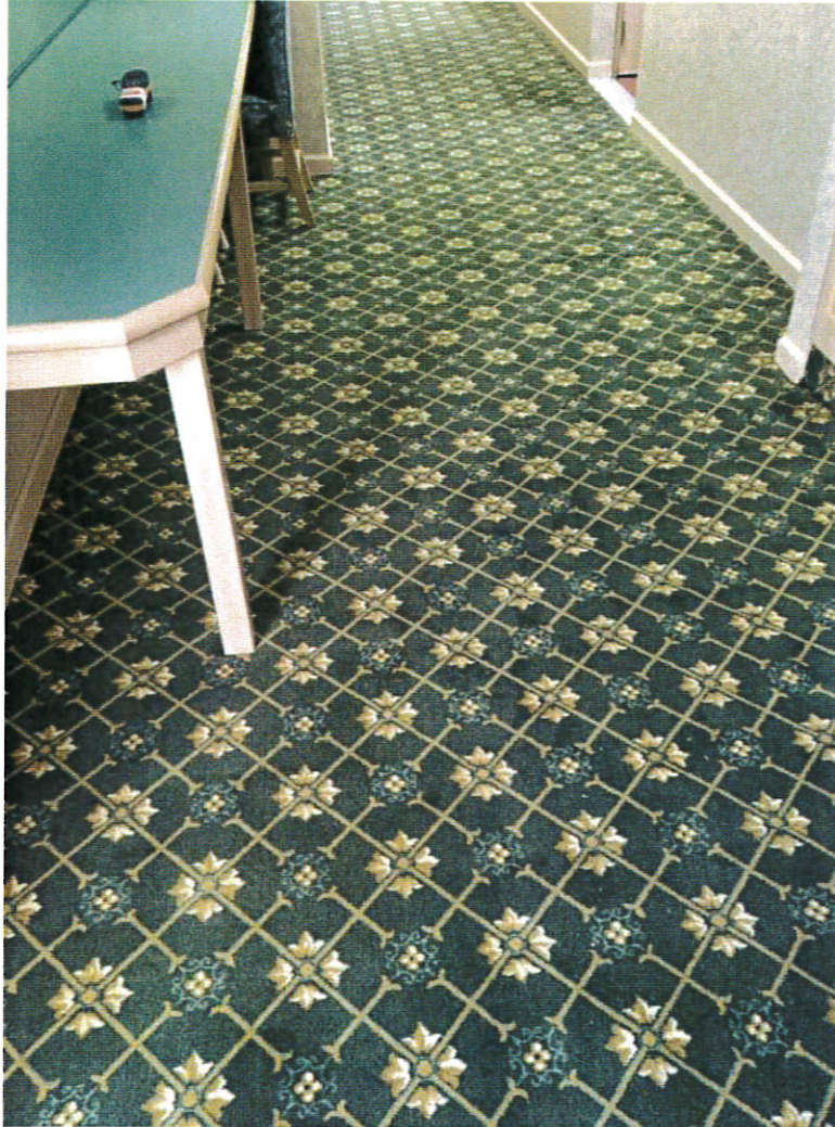
140 140-Pre-Mitigation - Locker room Date Taken: 12/26/2022 (Zone 1) 10
