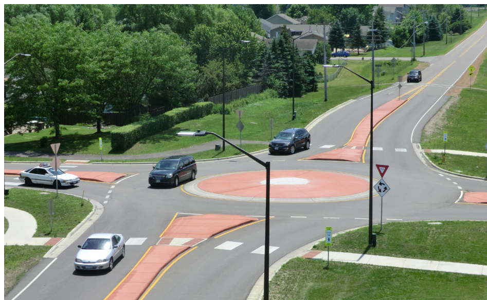
Example of a single-lane roundabout. Source: FHWA
