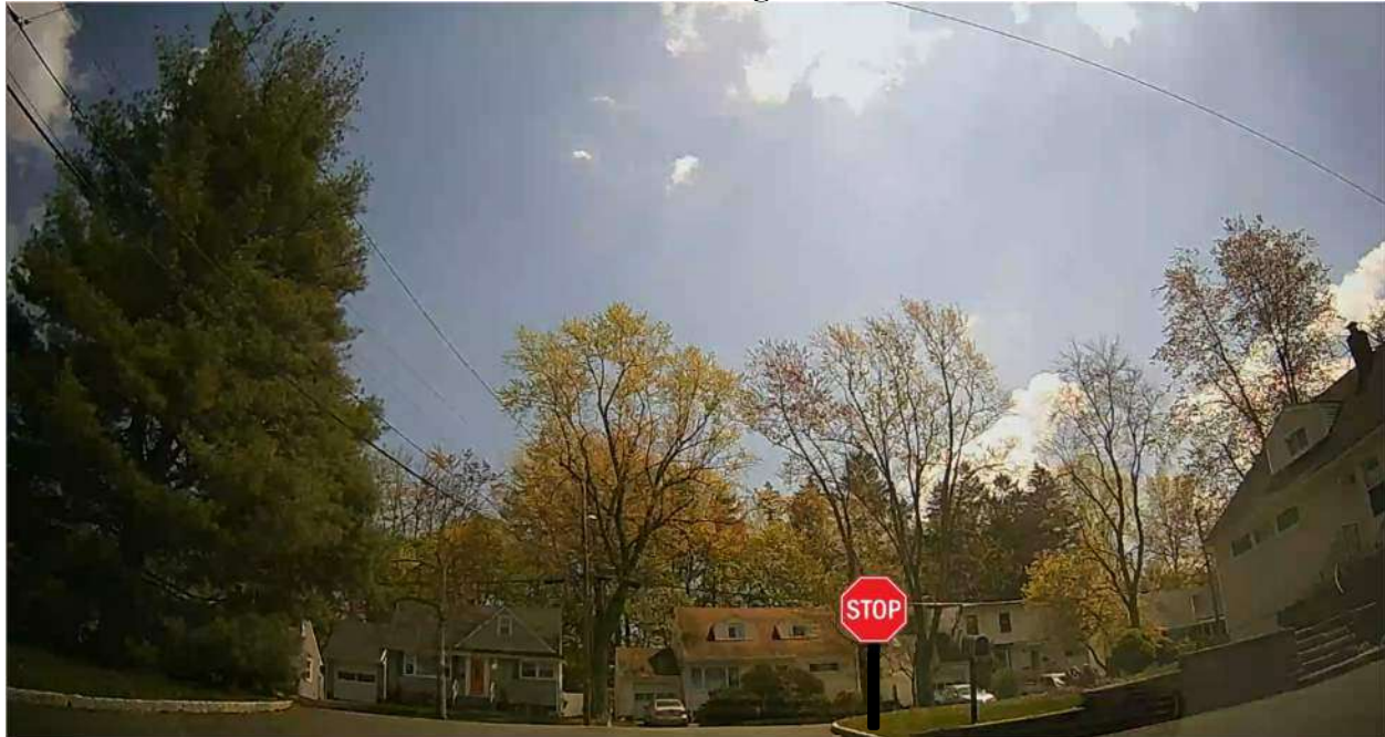
FIGURE 4 – STOP Sign Installation
