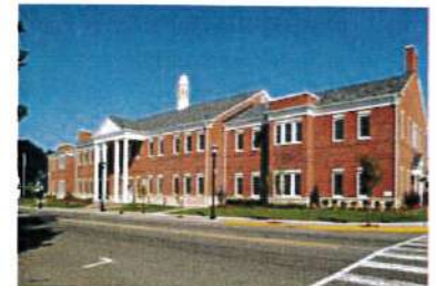
Hasbrouck Heights Municipal Complex
