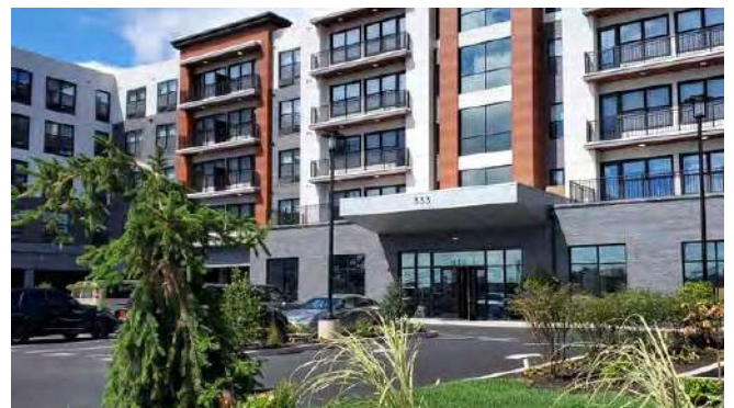
The Meadowside 333 Bergen Avenue Fairview, NJ
