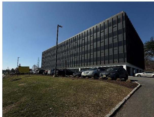
Figure 7: The property viewed from the northern driveway
