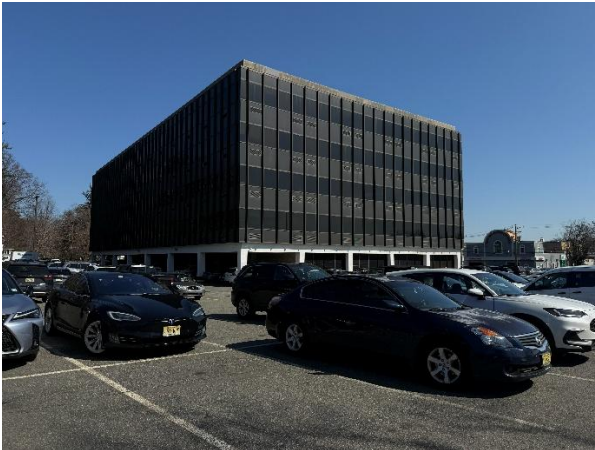
Figure 4: The office building viewed from the southern drive aisle
