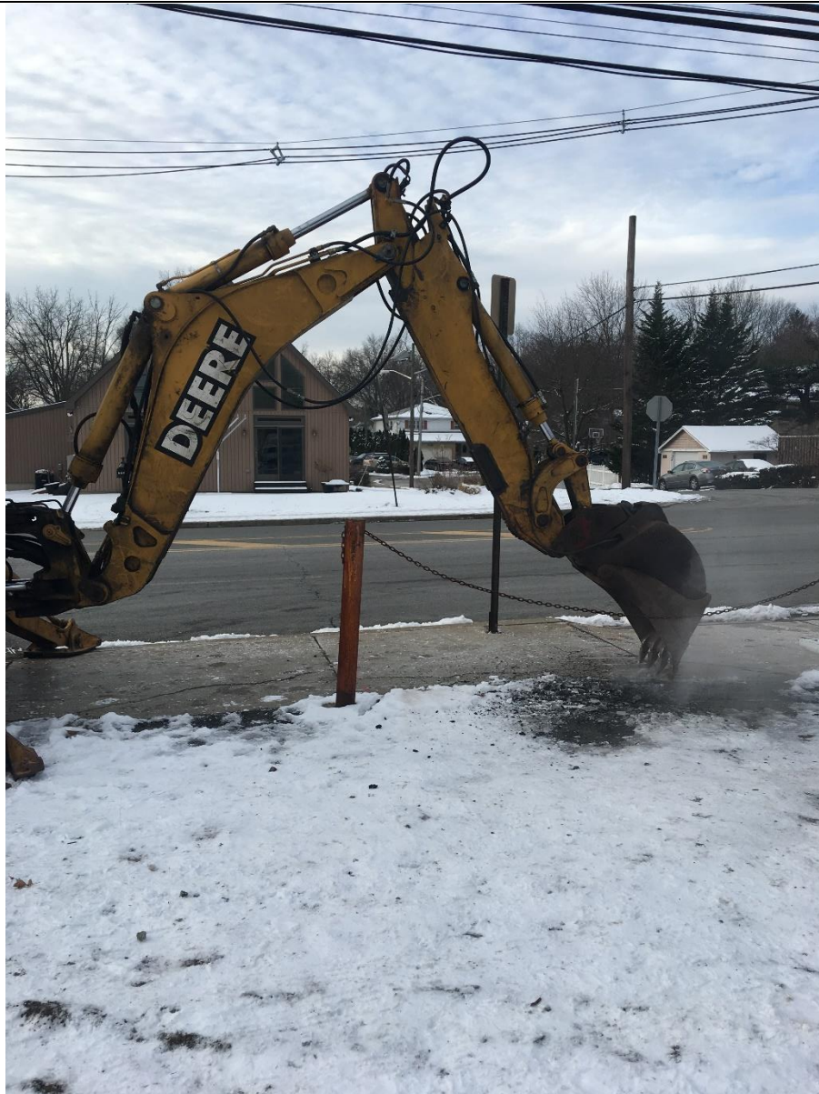
PHOTO 4: View of test pit location in the southwestern area of the Site.
