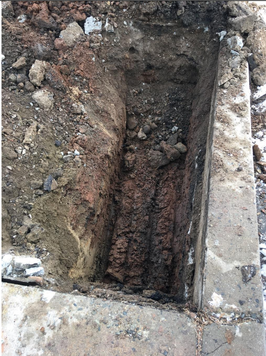
PHOTO 2: Looking east at south side of test pit located in the sidewalk along Eagle Rock Avenue (January 19, 2018).
