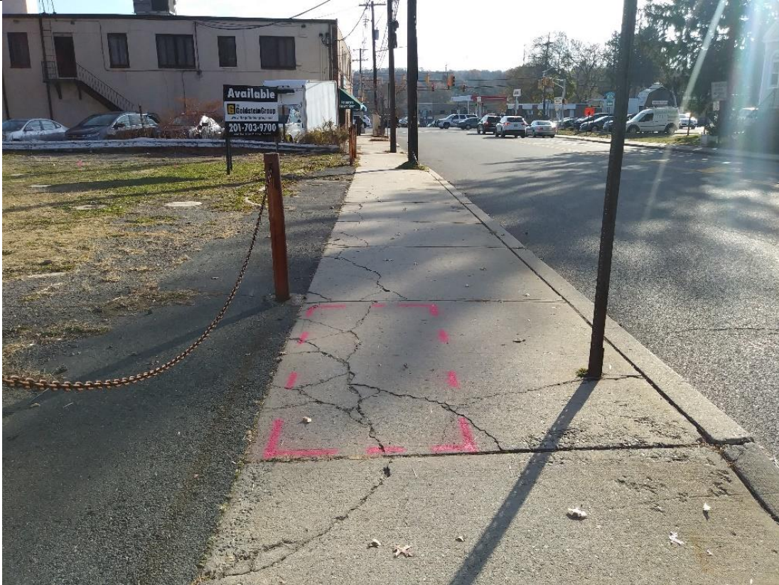
PHOTO 1: View of GPR anomaly (potential UST) located in the sidewalk near the southwest area of the Site (November 27, 2017).
