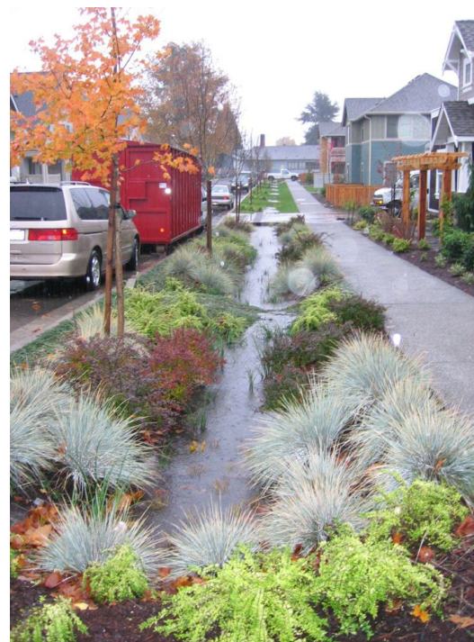
Bioswale example of stormwater best management practice
